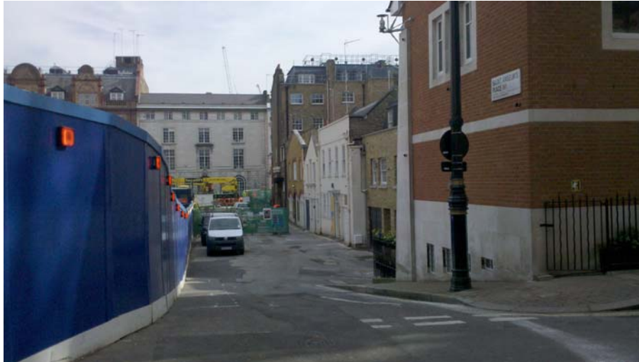
Plate 3: View from Gilbert Street looking east along St Anselm's Place: the topographic slope down towards the infilled channel revealed in Trench OAE1 is clearly apparent
