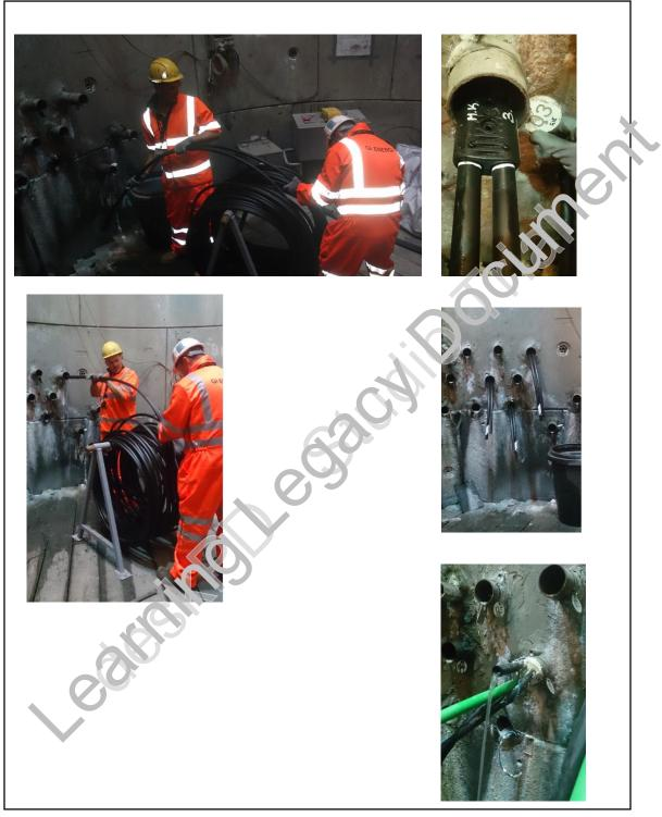
Figure 5: Installation of Loops into the TAMs
