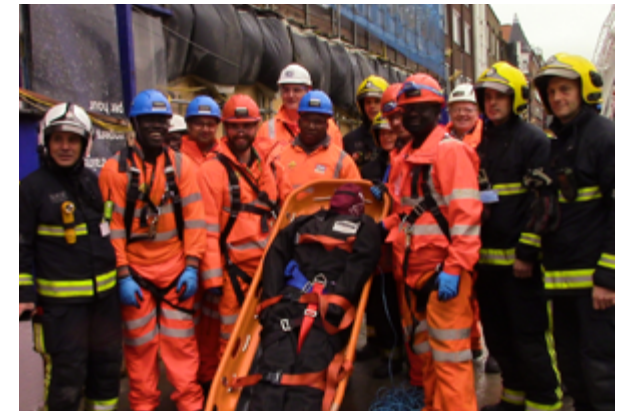
Emergency Crane Rescue at C422 Tottenham Court Road
