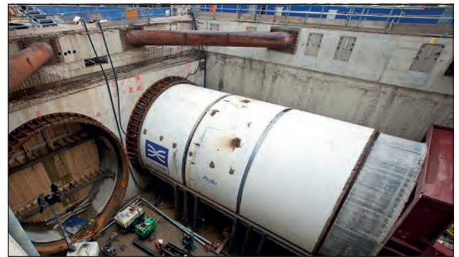
Figure 8. Drive X TBM launch on C300
