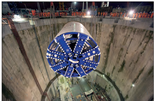
Figure 7. TBM cutter-head
