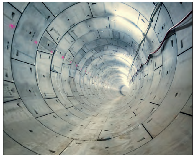
Figure 6. Completed section of segmentally lined running tunnel
