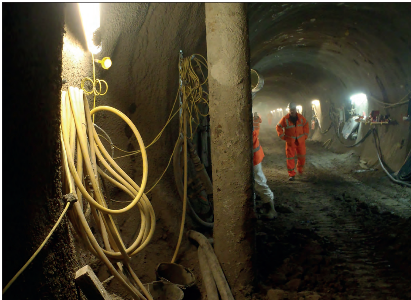
Figure 8. Steel-lined well in the grouting adit at Liverpool Street station
