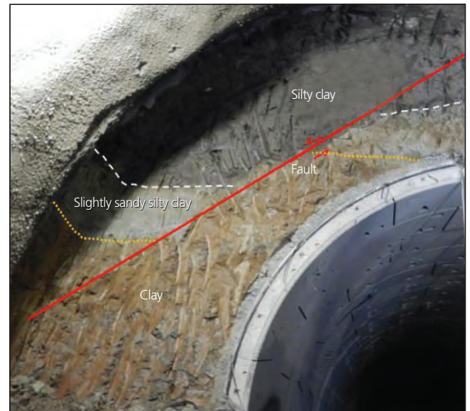
Figure 7. Faulted Lambeth Group strata at Farringdon station
