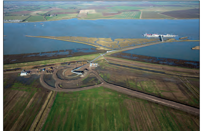
Figure 14. Half the 6Mt excavated material was used to create the Jubilee Marsh habitat creation project in Essex and part of the RSPB Wallasea Island Wild Coast Project – most of the rest was also beneficially reused
