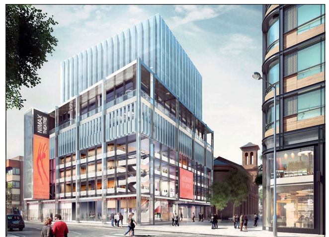
Figure 7. Tottenham Court Road Station eastern ticket hall – theatre oversite development
