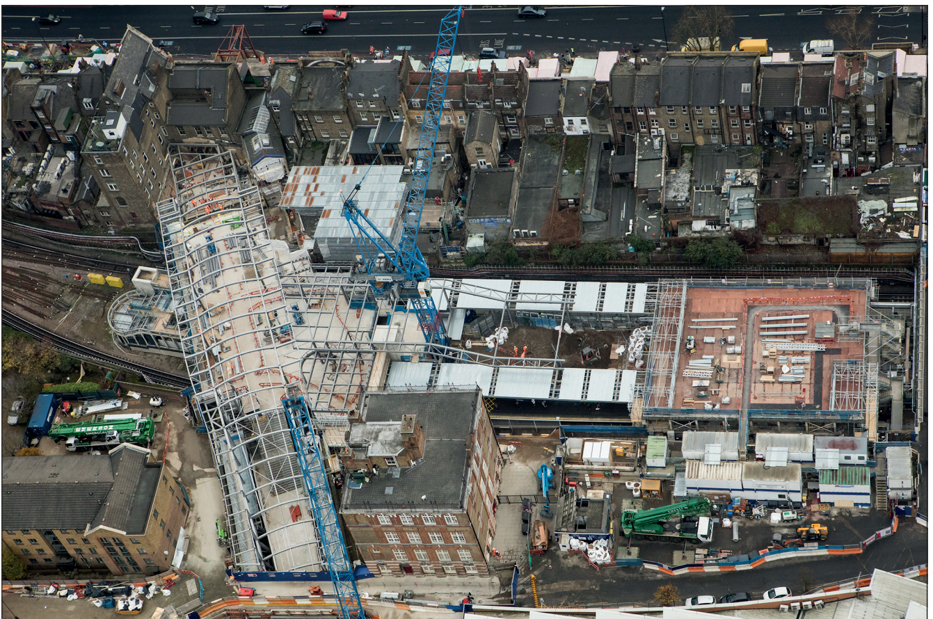
Figure 3. Whitechapel station: construction on a constrained urban site
