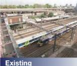
Crossrail's shallow cut and cover tunnels would occupy the space between Lord Hills Bridge and Ranelagh Bridge north of Royal Oak Station. An access road to the escape stair at the tunnel portal would provide access to this space. Following completion of work the area would be landscaped.
