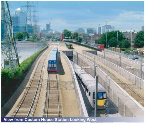
The two Crossrail lines would emerge from the tunnels with a new single track North London Line running between the Crossrail approach ramps.
