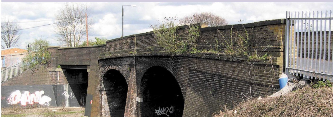
Church Lane / St Mary's Road Bridge
