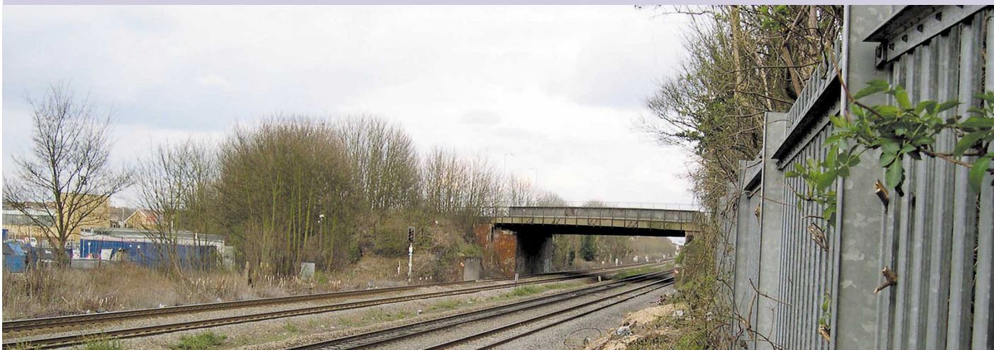
Uxbridge Road Bridge
