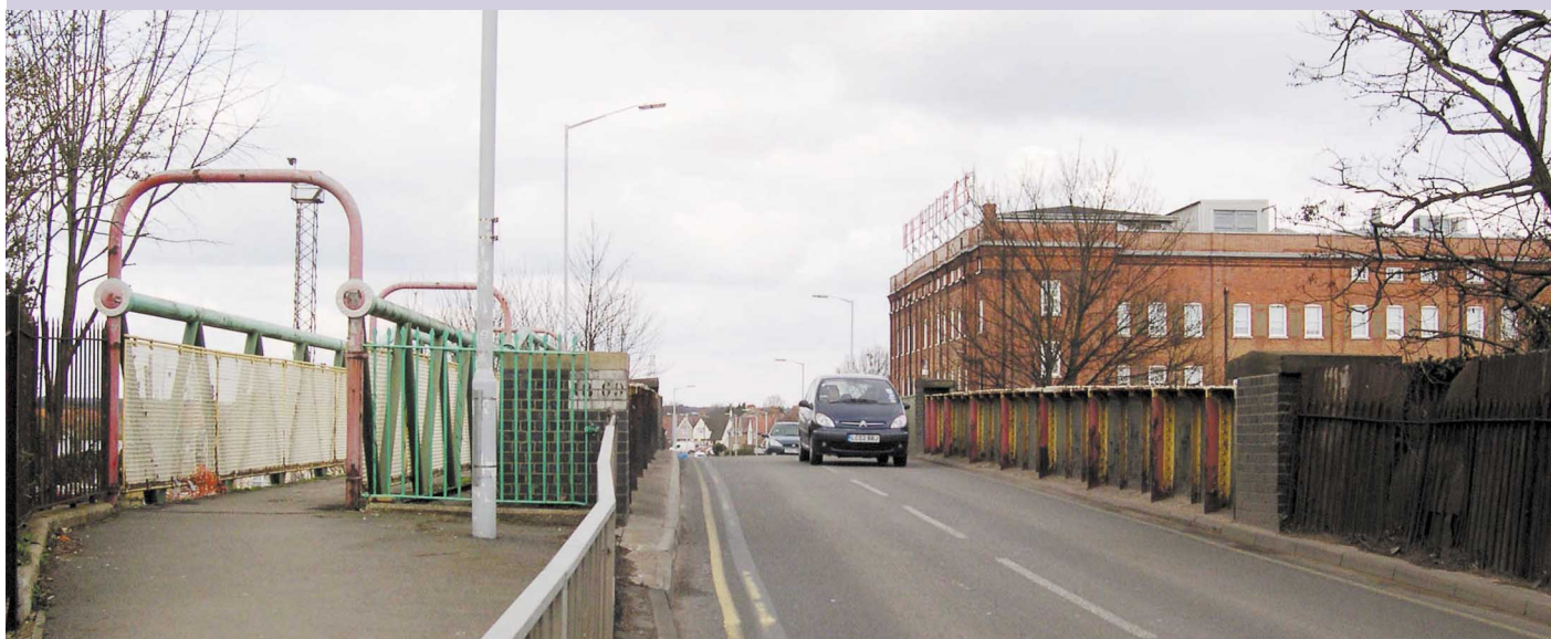
Stoke Poges Lane Bridge
