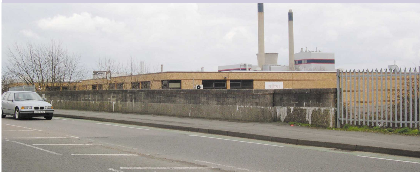
Dover Road Bridge
