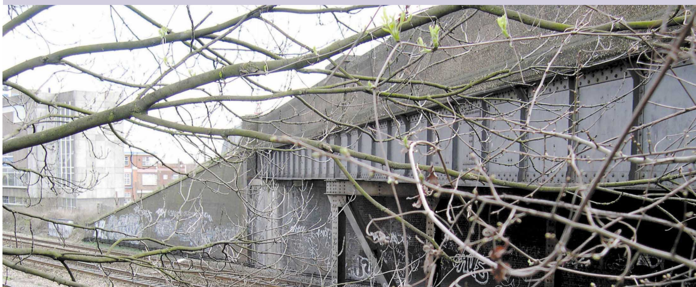
Farnham Road Bridge
