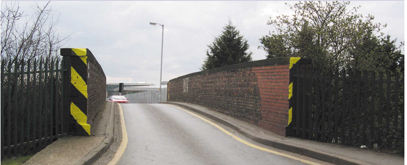
Leigh Road Bridge
