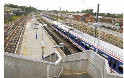
Acton Main Line station
