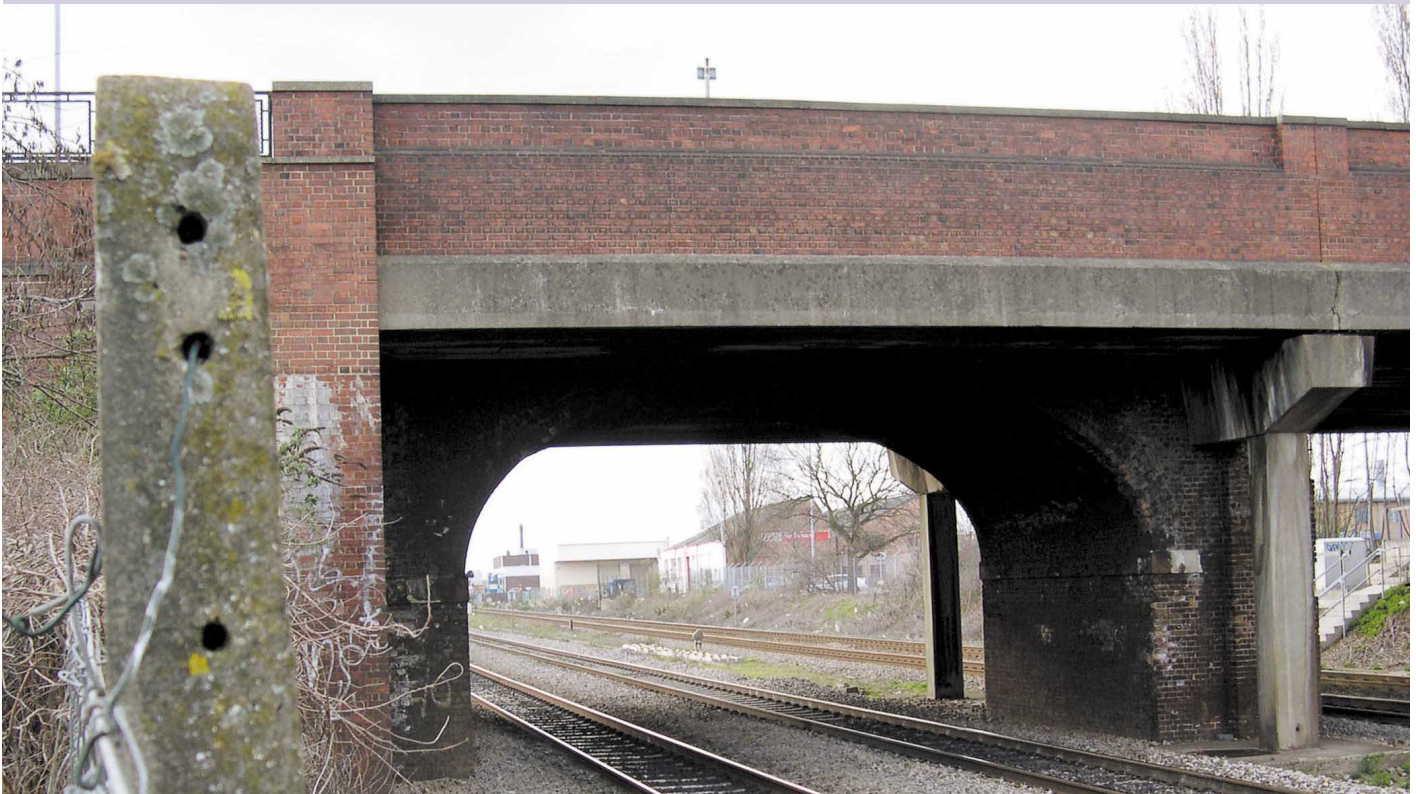
Wexham Road Bridge
