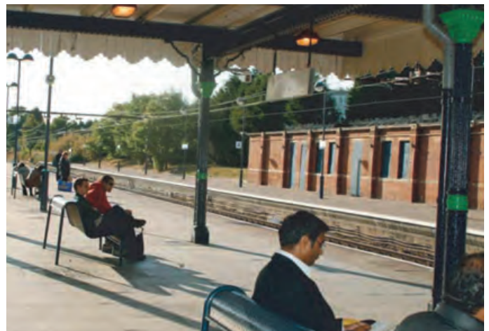
Seven Kings Station at present
