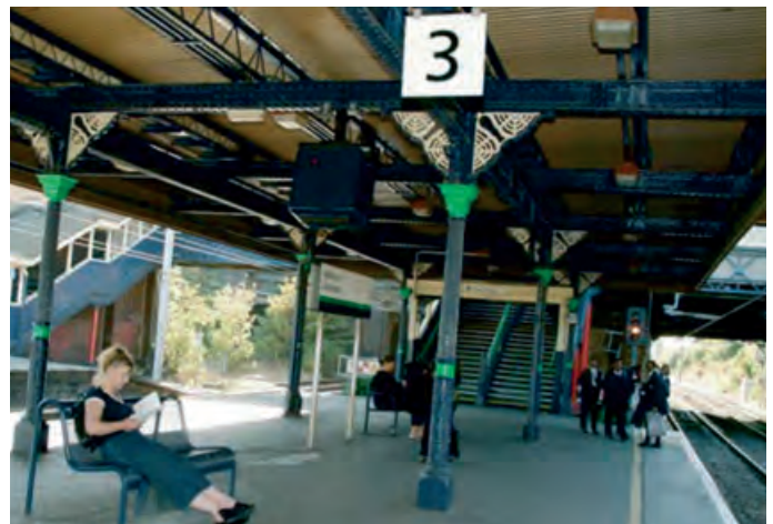
Goodmayes station at present
