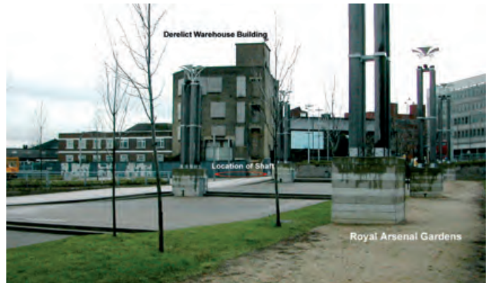
Warren Lane Shaft Site
