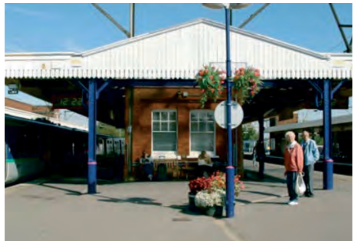
Shenfield station at present
