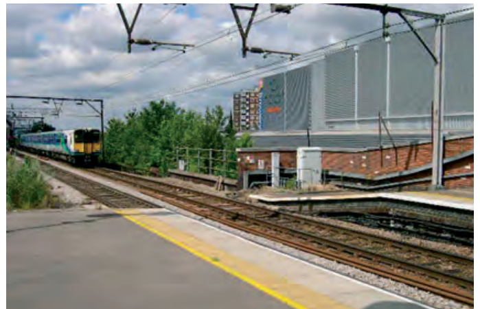
Romford station at present
