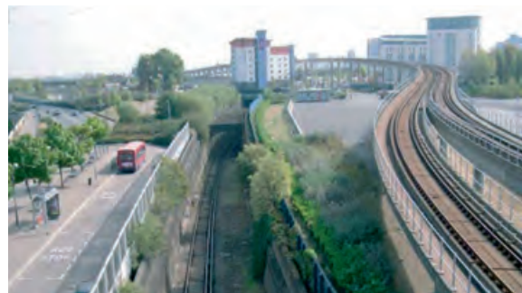
Connaught Tunnel at present
