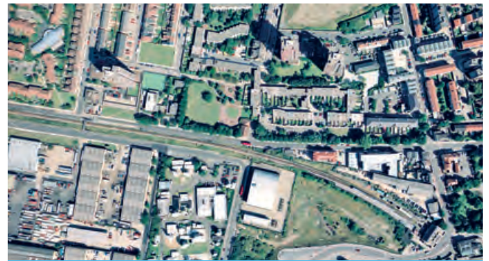
North Woolwich at present
