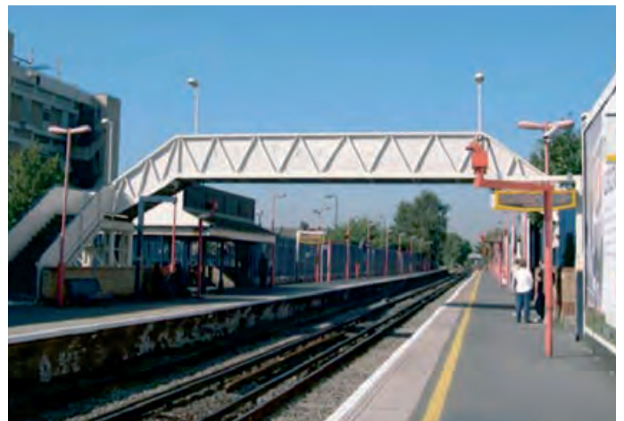
Abbey Wood Station at present
