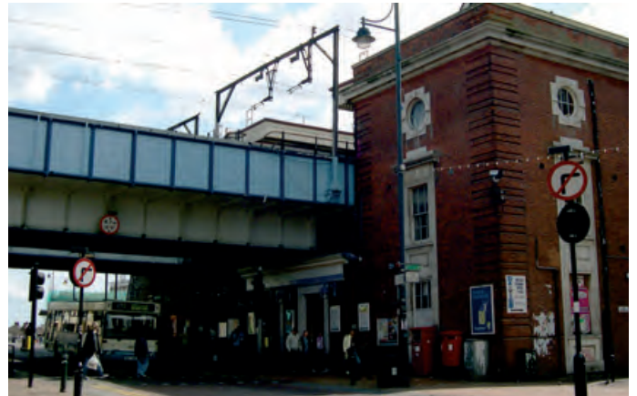
Romford station at present
