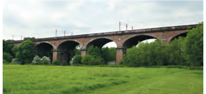
Wharncliffe Viaduct at present
