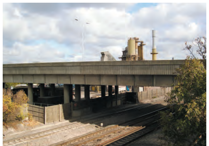
Stockley Road Bridge
