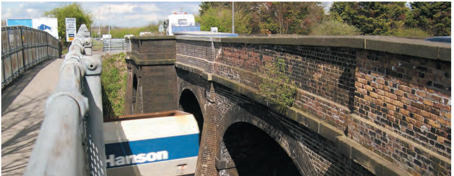
Thorney Lane Bridge at present
