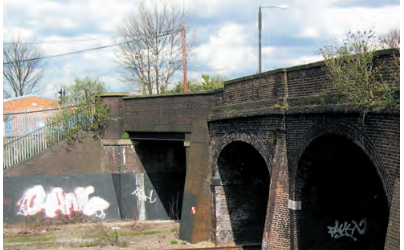
St Mary's Road Bridge
