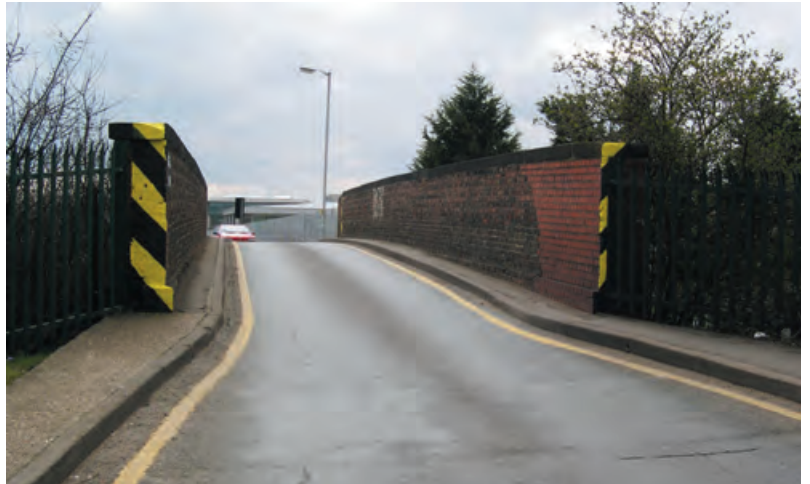
Leigh Road Bridge
