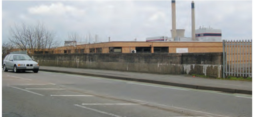
Dover Road Bridge
