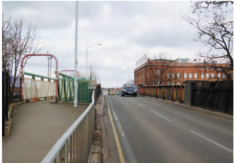
Stoke Poges Lane Bridge
