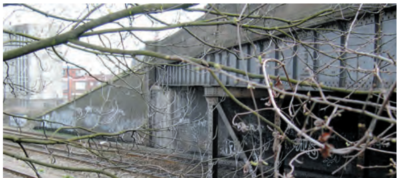
Farnham Road Bridge
