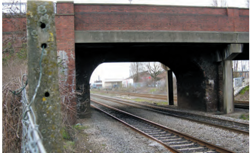
Wexham Road Bridge
