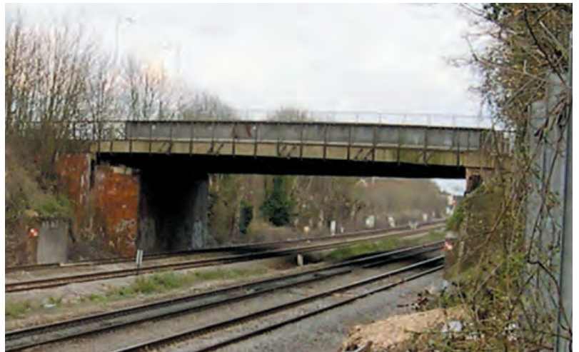
Uxbridge Road Bridge
