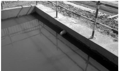
The site team estimates that the system allows them to recover up to a 1/4 of the water used to fill the sweeper water tank which equates to c.200litres of water recovered per catchpit discharge.
