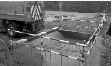
Photo 1 shows sweeper about to discharge into the catchpit:
