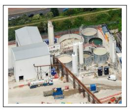
Above:Plumstead Slurry Treatment Plant, where recycled groundwater is used for slurry dilution.
