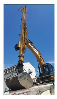
**Figure 7.** The innovation programme led to use of telescopic clamshell excavators on other projects following successful trials at Paddington, which found excavation rates increased from 48 m<sup>3</sup>/h to 54 m<sup>3</sup>/h
