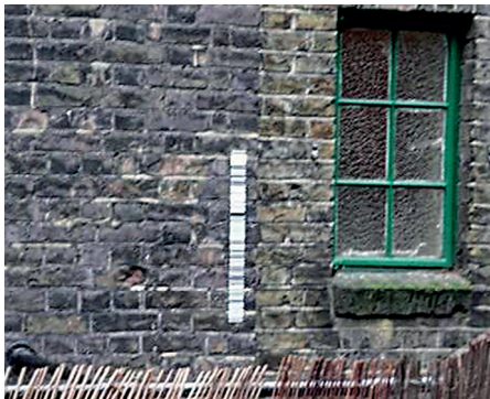
a) Invar scale on building facade – used for precise manual levelling
