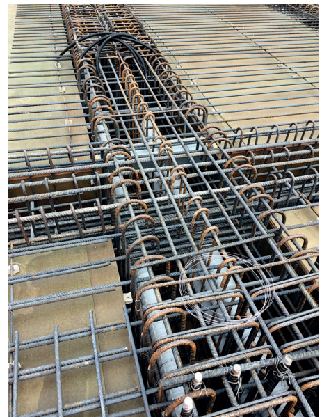
Figure 11 View of post-tensioned roof beams during installation of tendons
