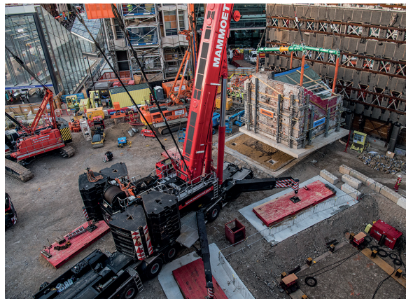
Figure 8 Smithy returned to original position in October 2017 by Skanska and Mammoet
