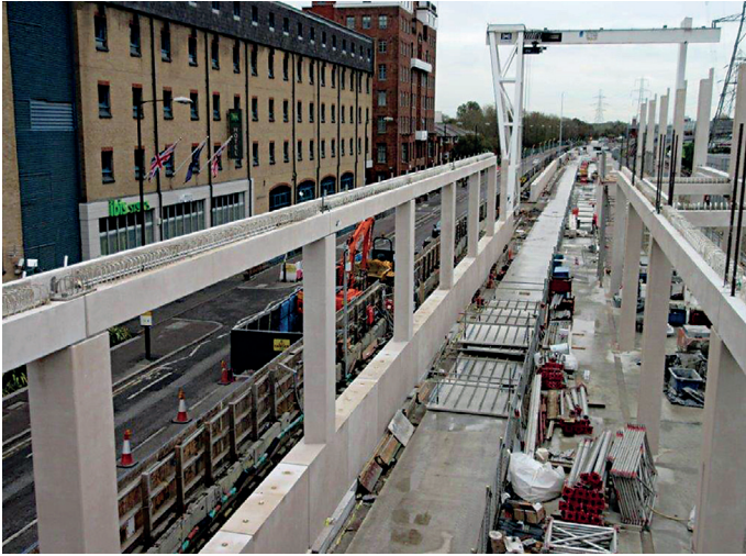
➔ Figure 14 Precast panels with triangular vaulted soffits are used on main span of concourse structure
