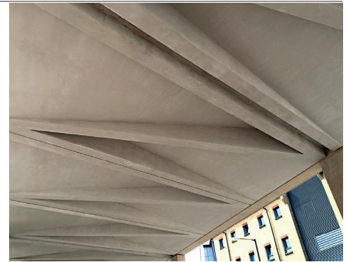
➔ Figure 14 Precast panels with triangular vaulted soffits are used on main span of concourse structure
