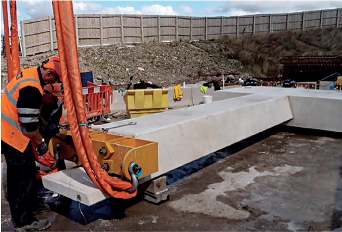
Figure 17 Victoria Dock Road column/ wall structures
