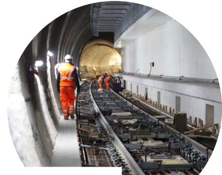
Underneath Soho and the Barbican, floating track slab has been installed to reduce the noise generated by the operational railway.
