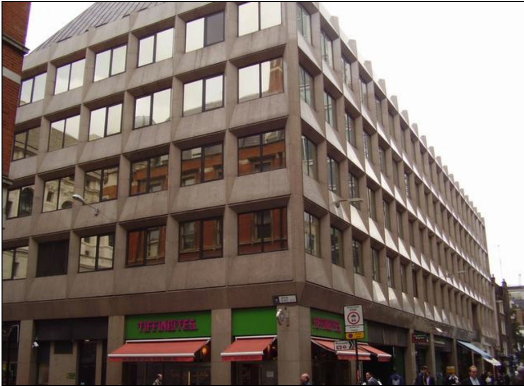
Plate 2: View of the assessment site and the former 101-109 Moorgate building from Moorfields looking southeast towards Moor Place
