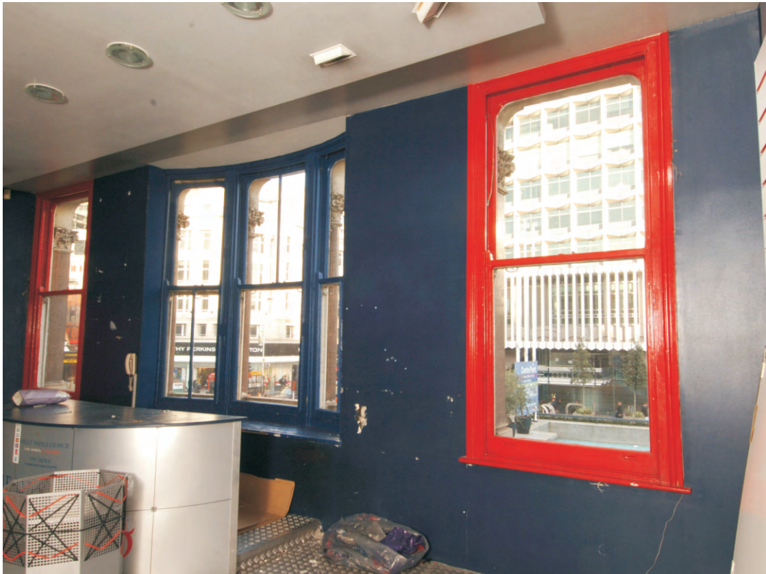
Fig 38 Interior of Building 3
