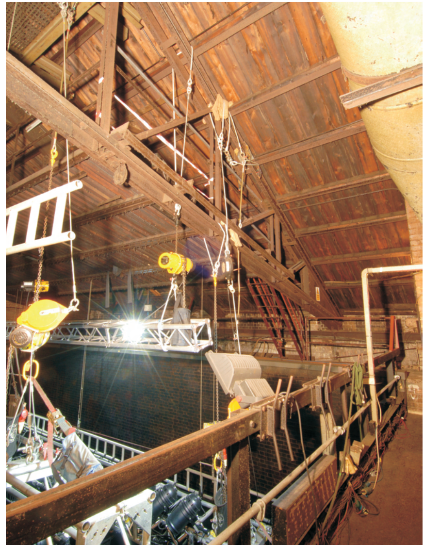
Fig 41 Walkways in roof space of Building 4
