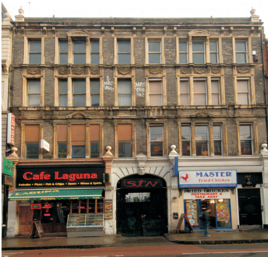
Fig 47 Exterior of Building 5
