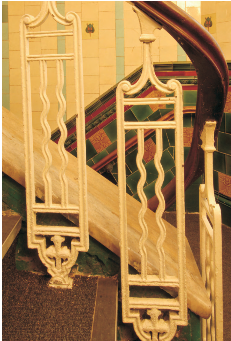
Fig 22 Cast iron balustrade in stairwell of Building 1
