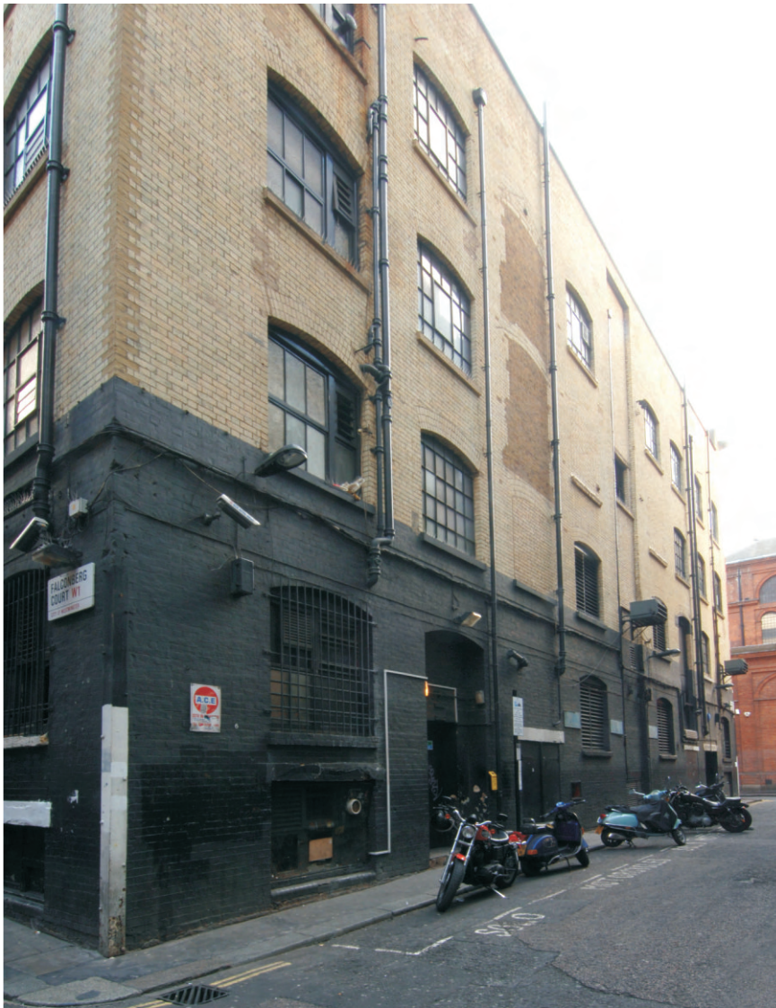
Fig 40 Exterior of Building 4 on Falconberg Mews
