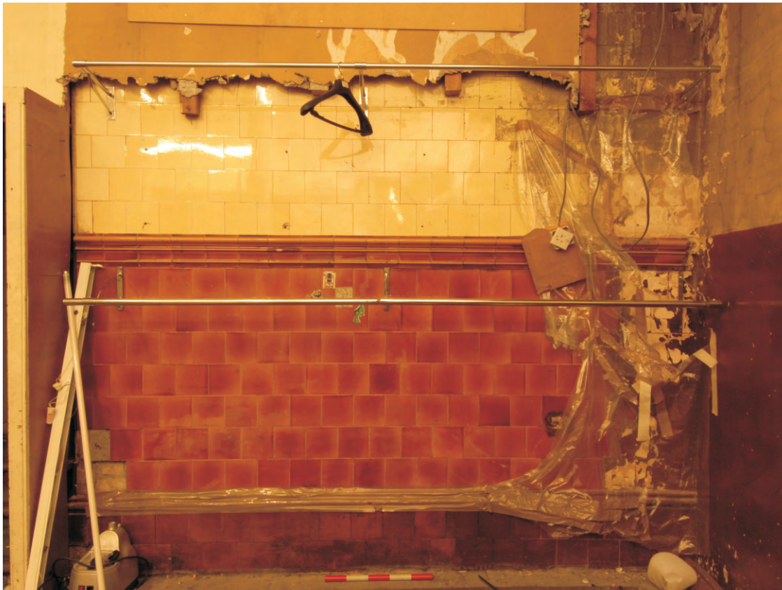
Fig 20 Tiles in rear ground floor room of Building 1
