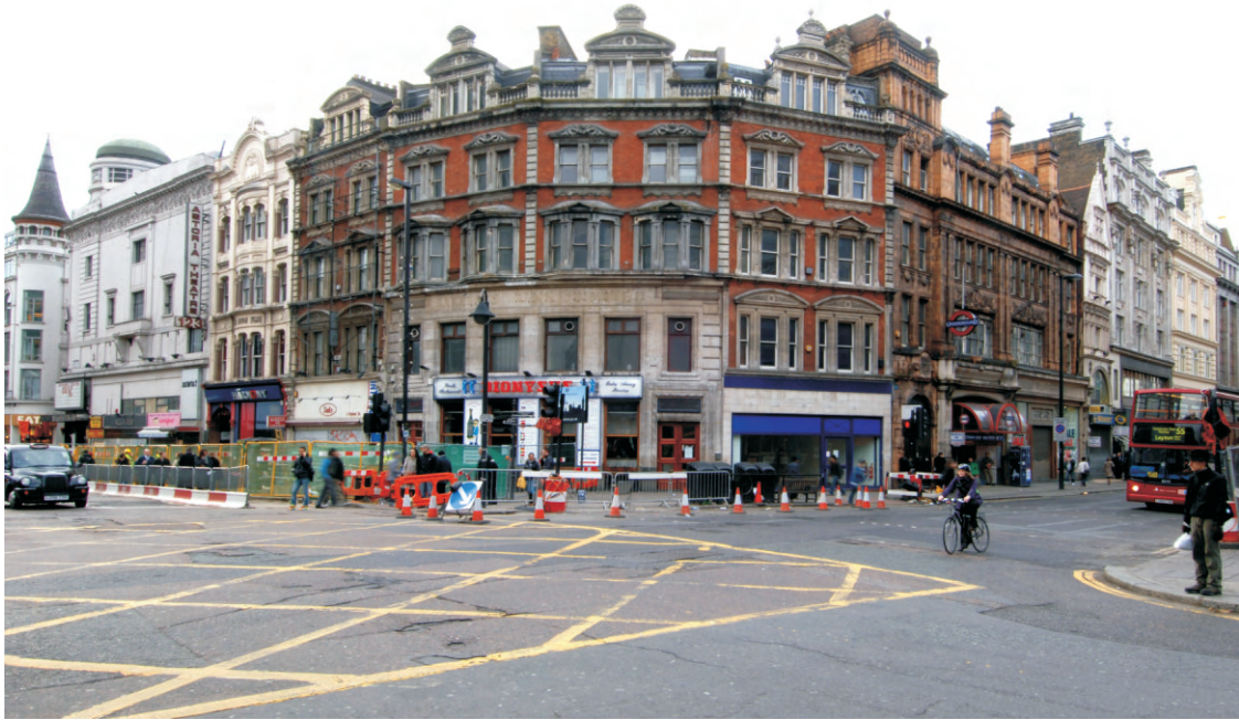
Fig 24 Exterior of Building 2
