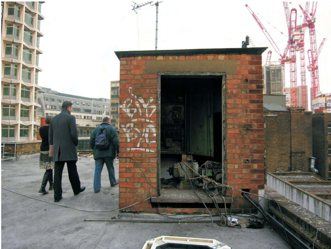
Fig 55 Square tower containing mechanism for goods lift in 144 Charing Cross Road
