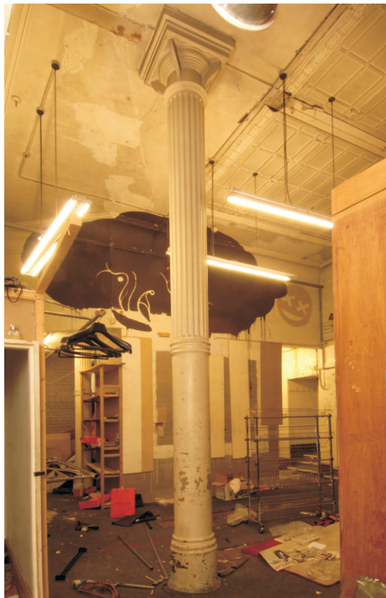
Fig 19 Cast iron column on ground floor of 9–15 Oxford Street
