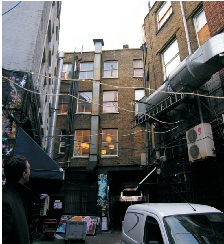
Fig 49 Rear of Building 5 facing south
