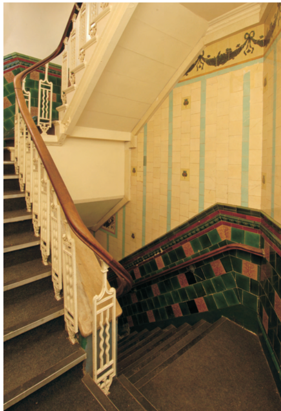
Fig 21 Tiles in stairwell of Building 1
