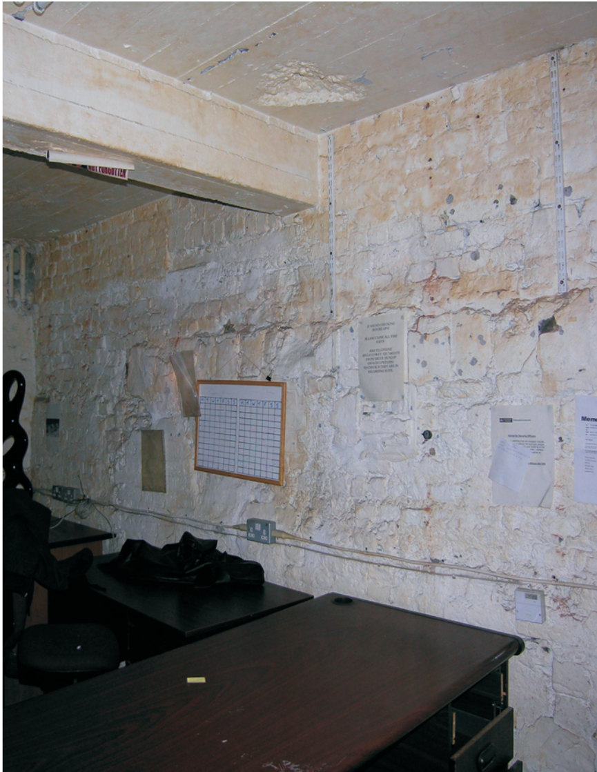
Fig 68 Multiphase wall in basement of 1-6 Falconberg Court
