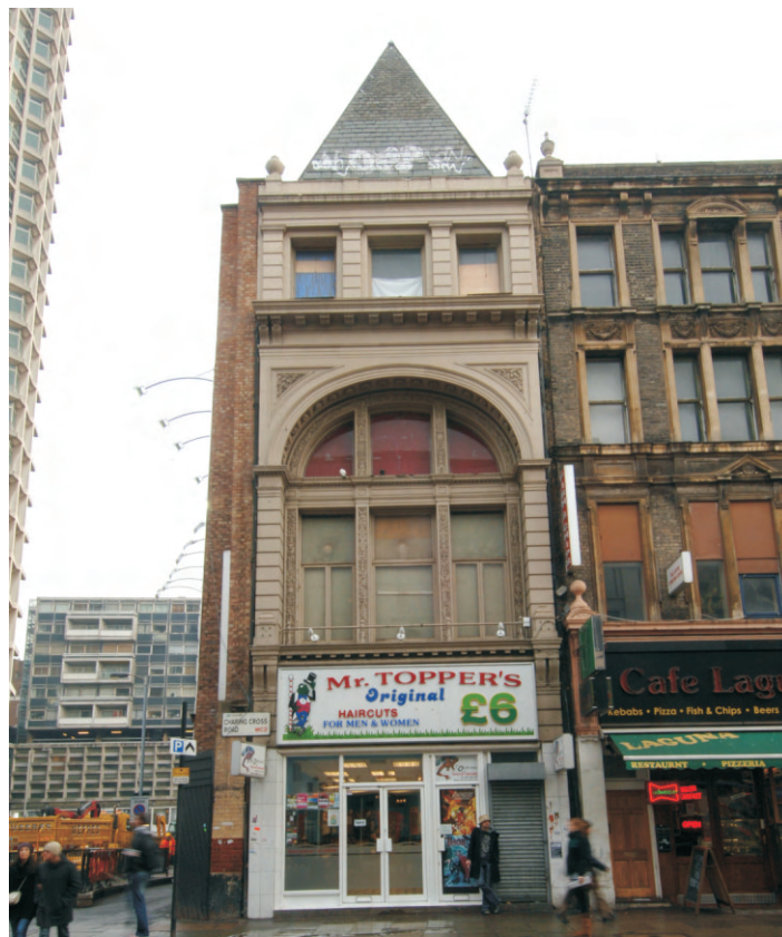
Fig 57 Exterior of 148 Charing Cross Road
