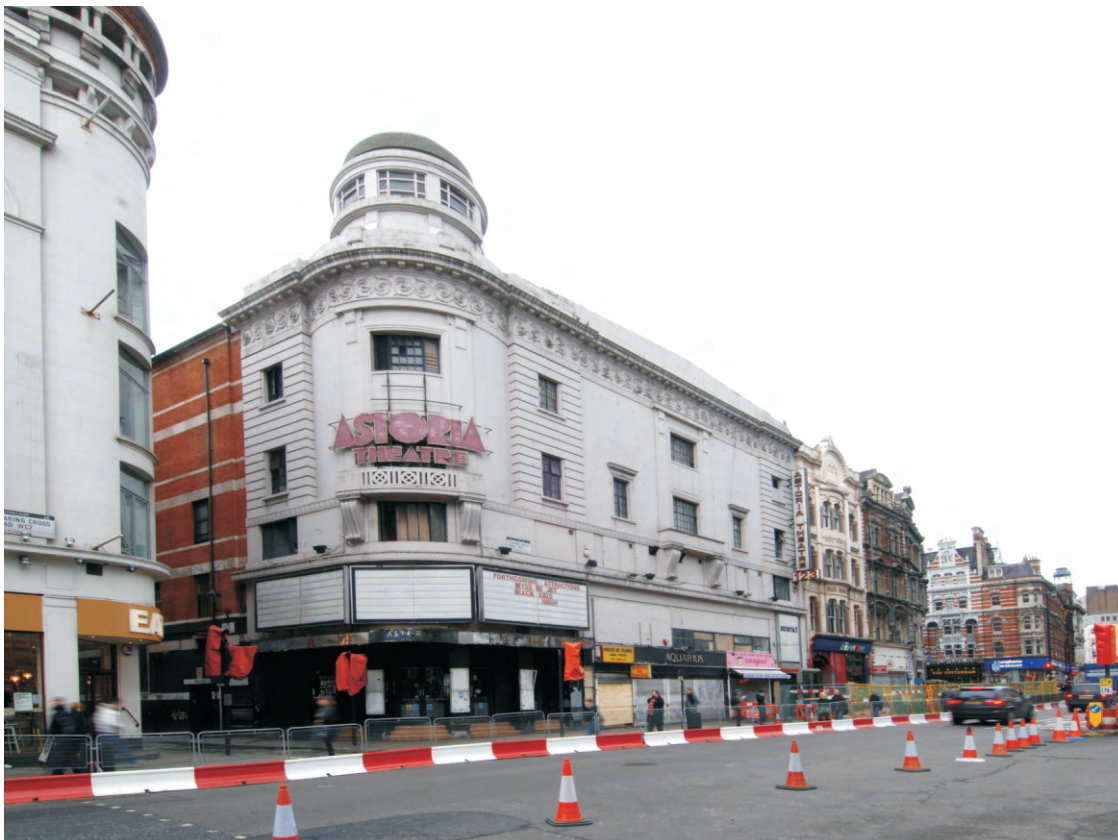
Fig 39 Exterior of Building 4 on Charing Cross Road
