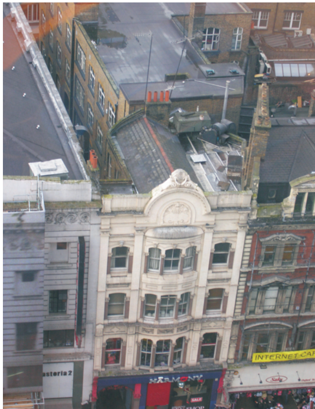
Fig 33 Aerial view of Building 3 showing roof and chimneys
