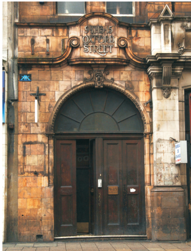
Fig 17 Arched entrance to upper floors of 9-15 Oxford Street showing inscription
