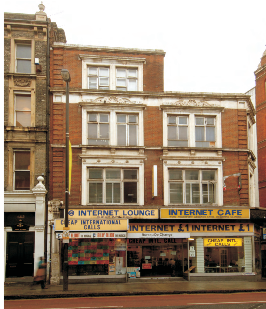
Fig 63 Exterior of Building 7 facing onto Charing Cross Road
