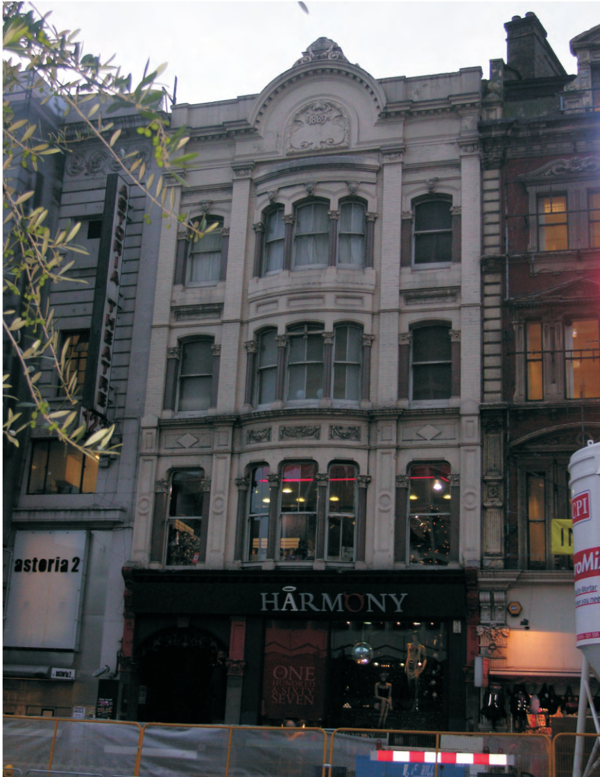
Fig 34 Exterior of Building 3
