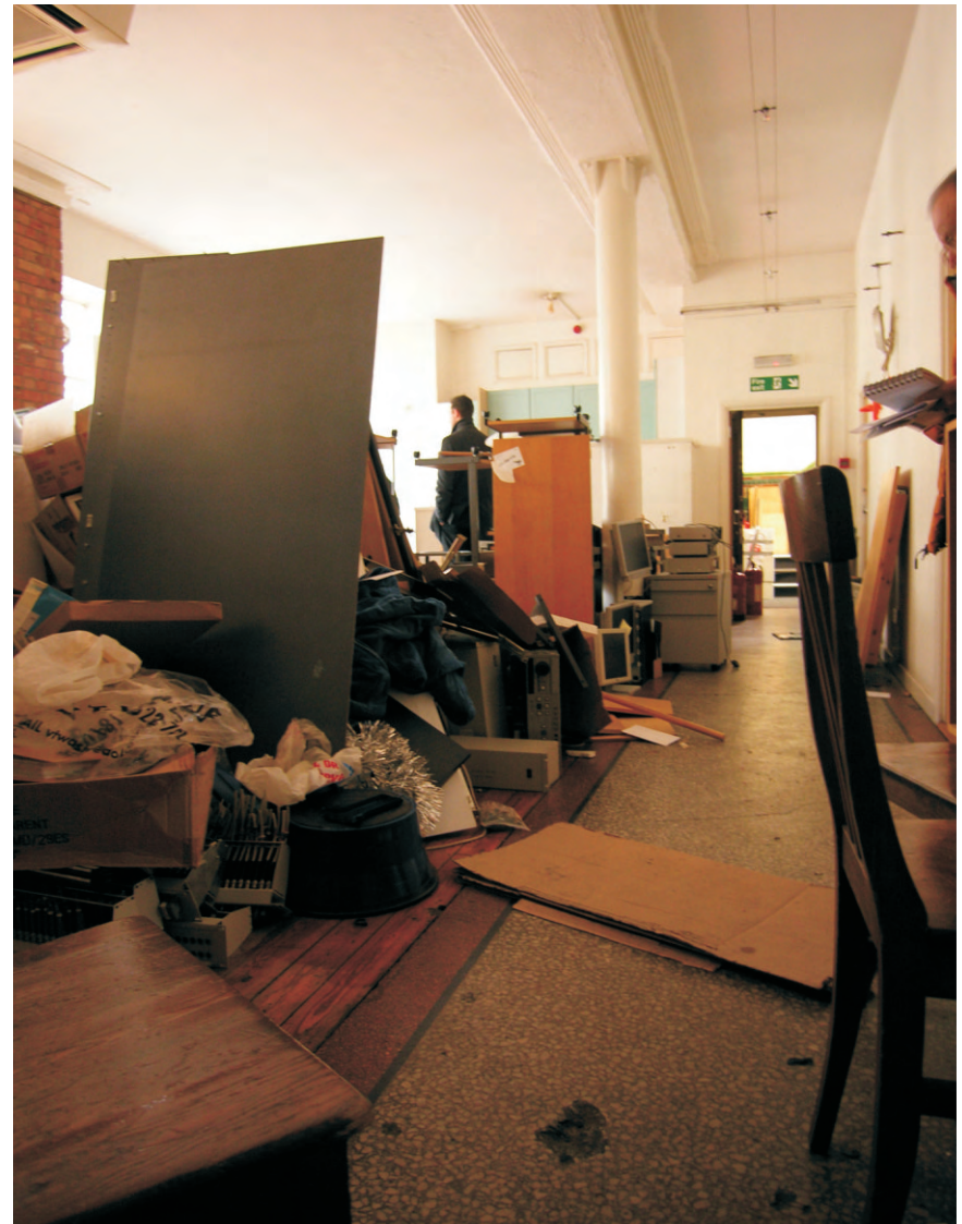
Fig 23 Mosaic corridor and undecorated columns on first floor of Building 1
