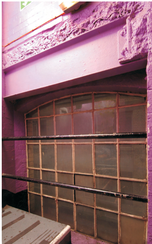
Fig 43 Adapted window opening for insertion of stairs
