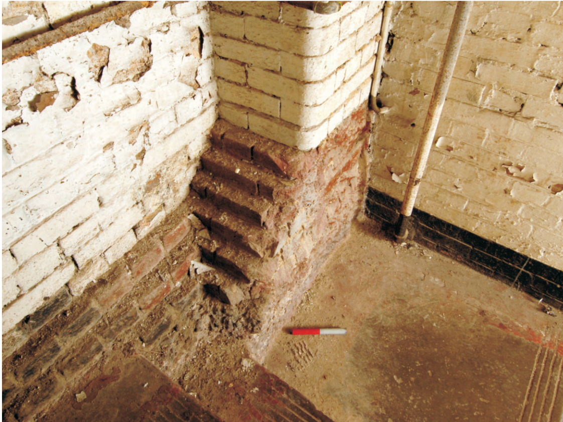
Fig 42 Cut-back stepped brick wall footings in south-west corner of Astoria 1
