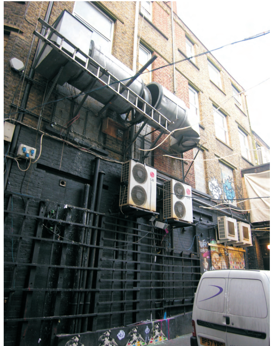
Fig 53 Exterior of 144 Charing Cross Road
