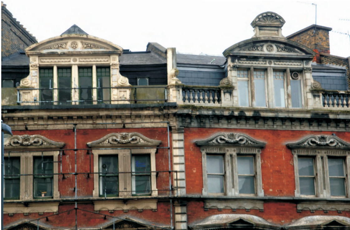
Fig 25 Dormer windows of 1 and 3 Oxford Street
