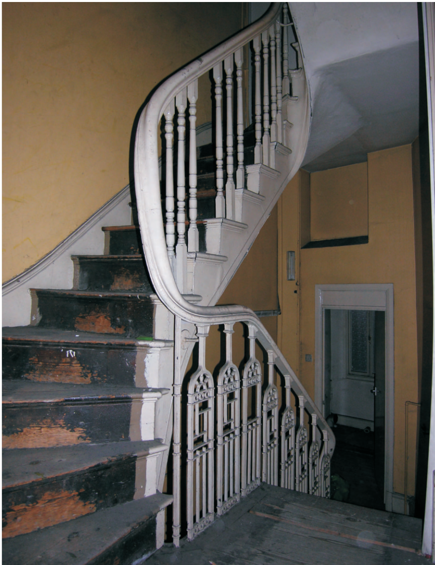
Fig 26 Art deco cast iron balustrade of staircase in 1 Oxford Street
