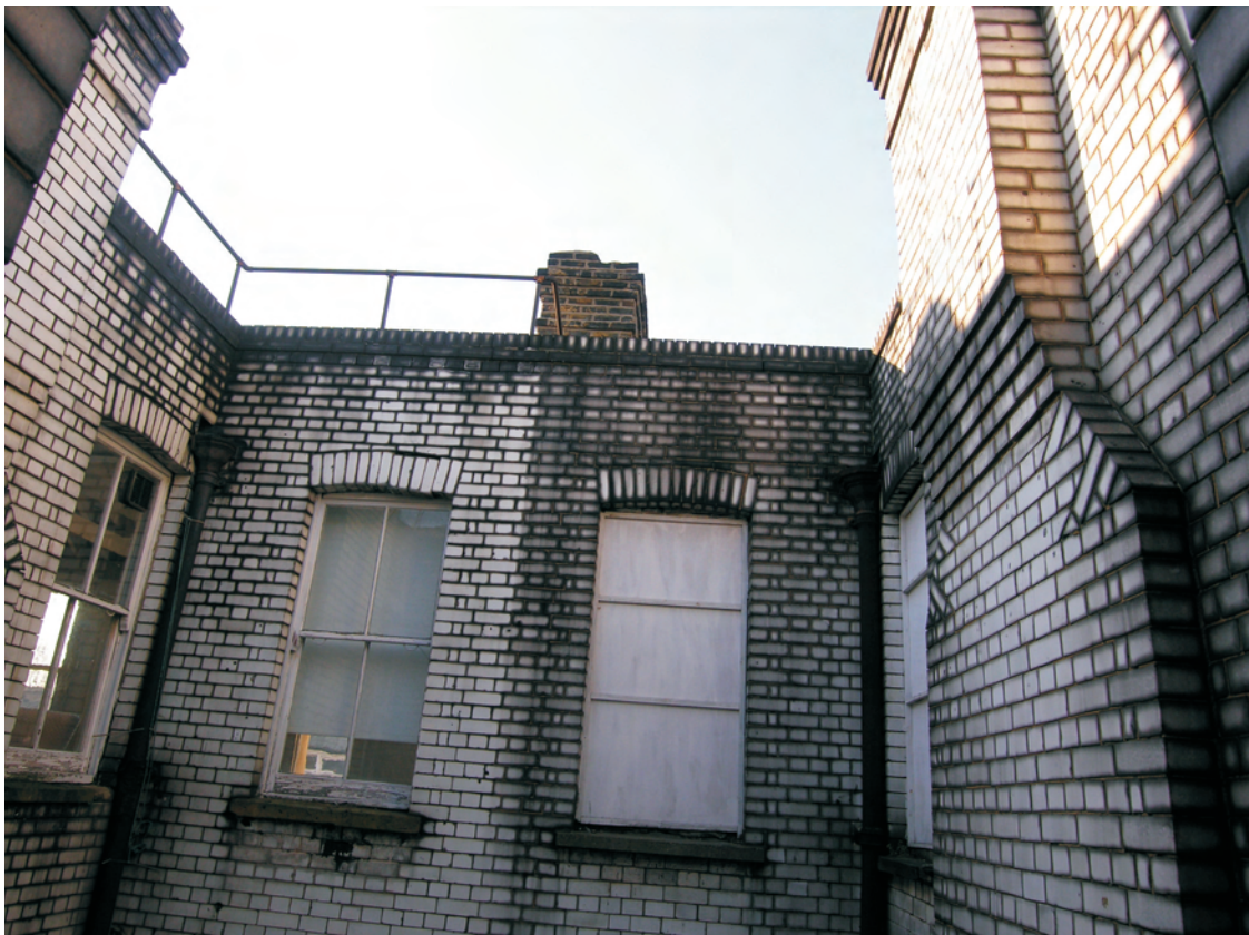
Fig 51 Brick chimney stacks in internal light-well in Building 5
