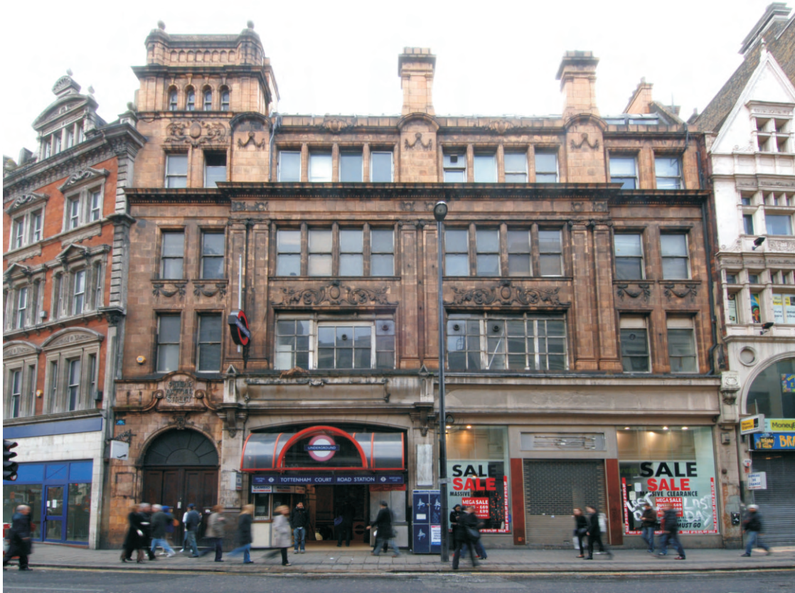
Fig 16 Exterior of Building 1
