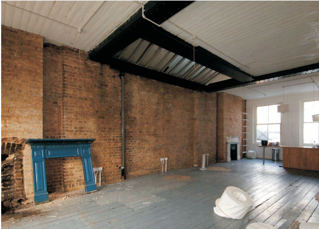
Fig 50 Interior large room in Building 5
