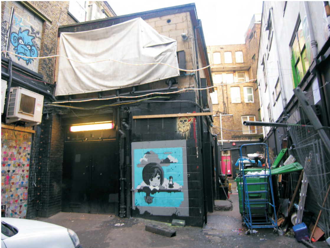
Fig 54 Concrete block extension to 144 Charing Cross Road
