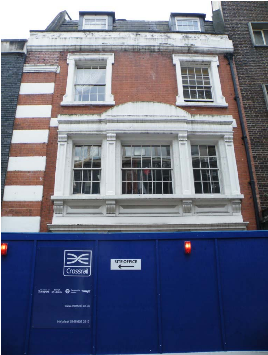
Plate 1 General view of the façade
