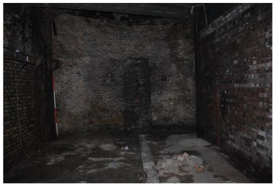
Plate 67- Vault showing exposed brickwork and buttress
