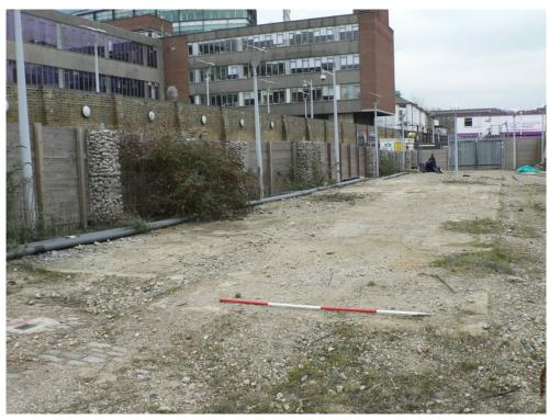
Plate 7 – Upper Triangle site showing concrete base to former police station and granite setts to front of photograph
