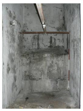
Plate 30 – Concrete lined western section of vault one, note corbel to left and horizontal buttress to rear
