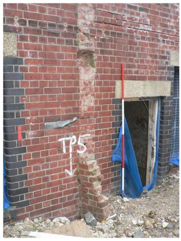
Plate 18 - Detail of former partition to brick vaults outside Vault 3
