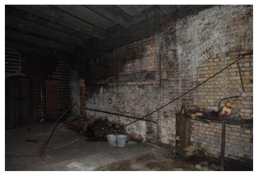
Plate 70 – Western elevation of vault, showing straight joint of wall to centre and change of floor level suggesting the room was originally divided into two.
