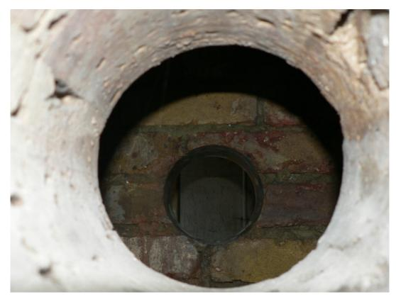
Plate 40 – Core hole showing blocked niche was originally hollow
