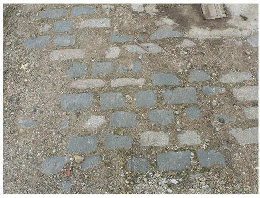
Plate 5 – Granite setts located on Upper Triangle site
