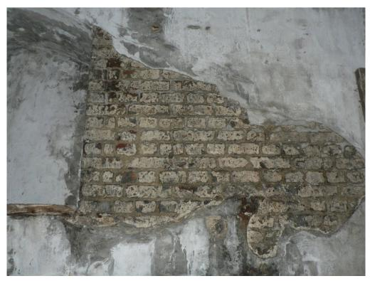
Plate 60 – Exposed brick work showing English Bond
