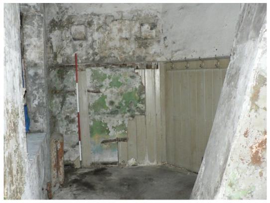
Plate 63 – Vault with surviving wood panelling and coat hooks
