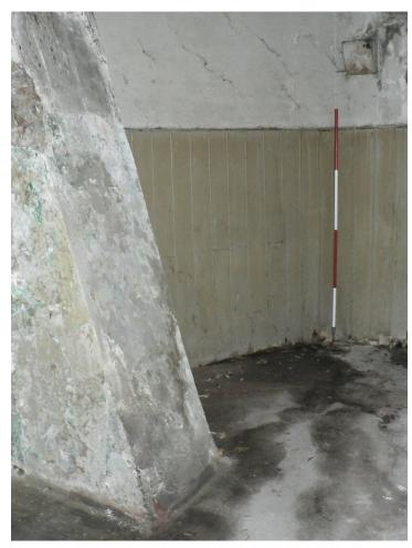
Plate 64 – Concrete rendered buttress and panelling
