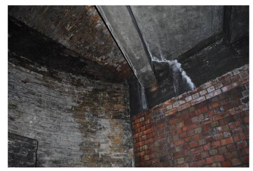
Plate 73 – Ceiling detail showing inserted concrete frame
