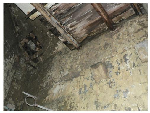
Plate 50- Ceiling detail showing chimney flue and corbels
