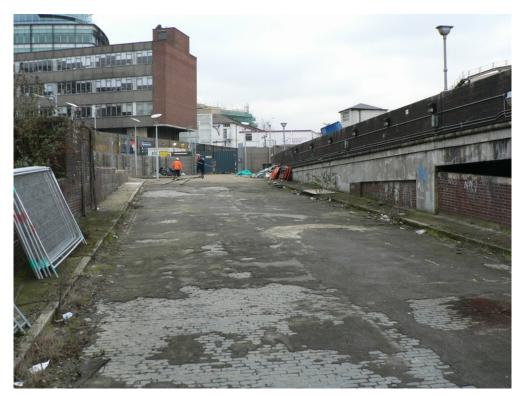
Plate 10 – View up Goods Ramp showing historic granite sett partially covered by tarmac
