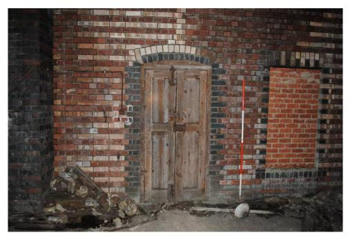
Plate 72 – Opening to track side and bricked up aperture
