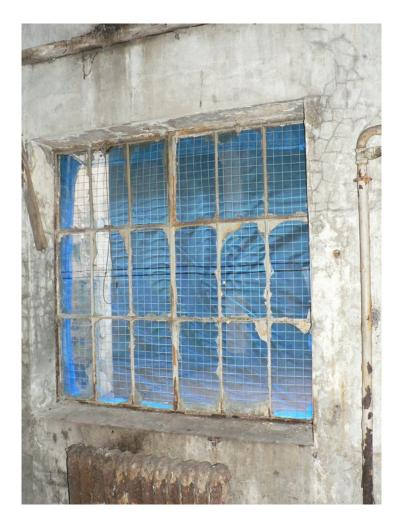
Plate 62 – Typical window detail, here with 18 panes
