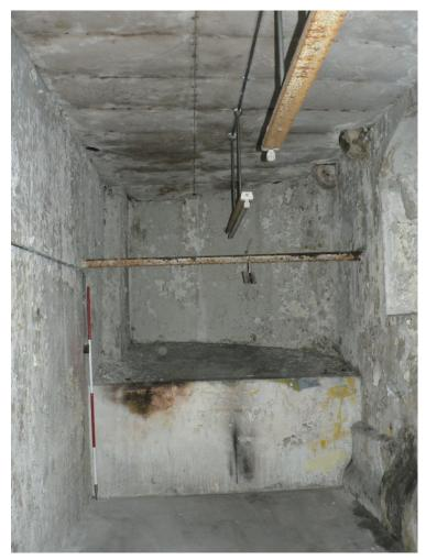
Plate 46- Obscured brackets, note corbels supporting roof above
