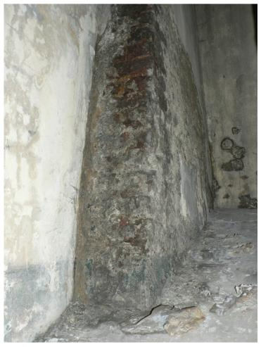
Plate 54 – Part of brick buttress obscured by partition wall
