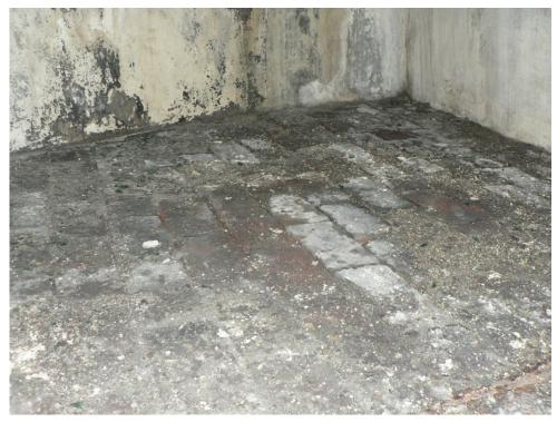
Plate 49 - The only vault to have exposed paviers to vertical buttress surround
