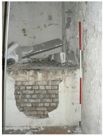
Plate 43 – Exposed brickwork in English Brick Bond
