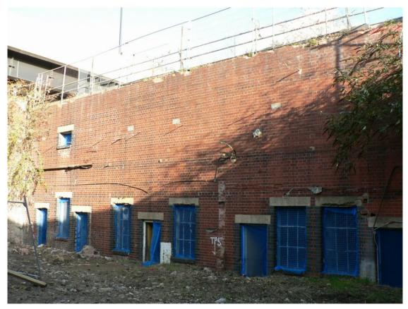
Plate 17 – Facade of refaced and truncated brick vaults
