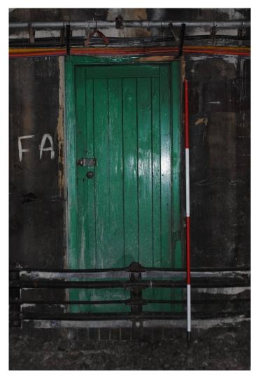
Plate 83 – Plank and batton door from trackside
