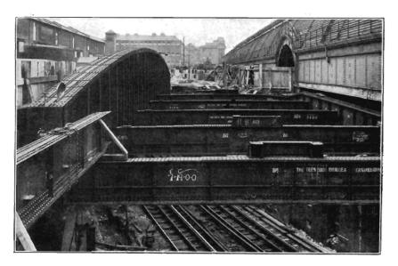
Plate H: Photo of showing bow string girder over the Bishop's Road tunnel at the west end of the London Street Deck
