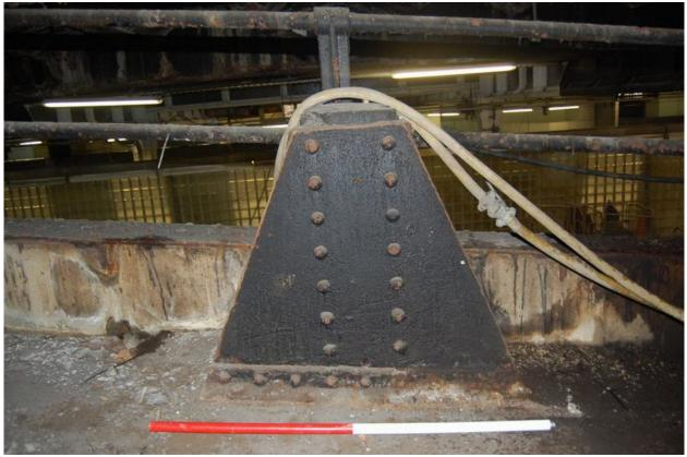
Plate 11: west elevation of inverted stanchion on ramp
