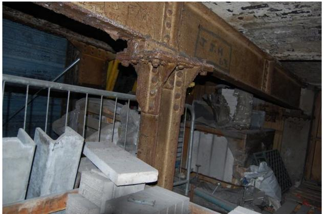
Plate 57: Central stanchion within office space – west elevation
