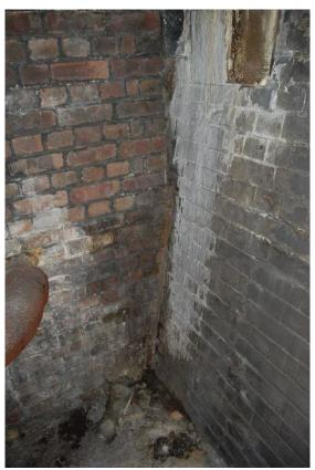
Plate 10: Junction between retaining wall and petrol inceptor
