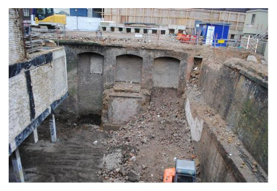
Plate 155 - Chimney and retaining walls, note void at intersection where chimney has been demolished
