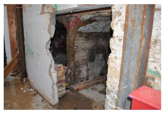
Plate 73 - 20-23 Long Lane and 22 Lindsey Street, vault detail post demolition
