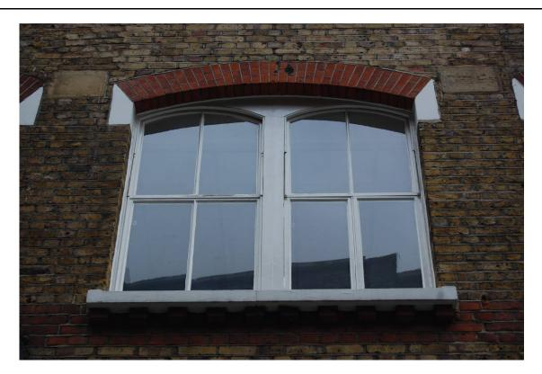
Plate 34 - 8-9 Hayne Street, inserted window after removal of walkway. Note stones either side of lintel
