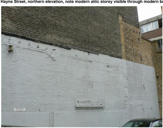
Plate 36 - 8-9 Hayne Street, showing blocked up apertures that used to lead into 10 Hayne Street, note also scarring to right of photo showing former roof over railway sidings
