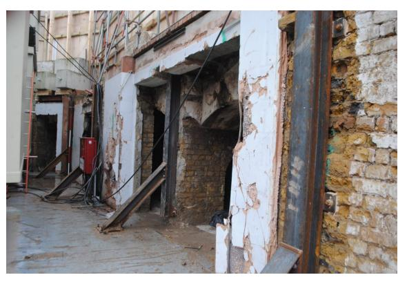
Plate 71 - 20-23 Long Lane and 22 Lindsey Street, vault detail post demolition
