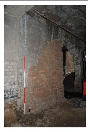
Plate 126 - 3 Lindsey Street, partially blocked archway that originally provided access to sidings
