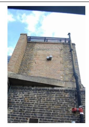
Plate 39 - 8-9 Hayne Street, view to rear, blocked up door that previously housed a bridge to 2 Lindsey Street
