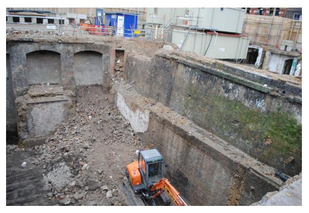
Plate 154 - Chimney and retaining walls, note void at intersection where chimney has been demolished
