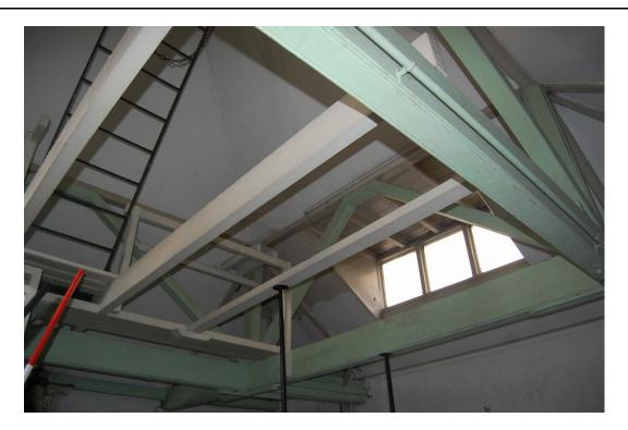
Plate 145 - 3 Lindsey Street, fink trusses and lights to roof above
