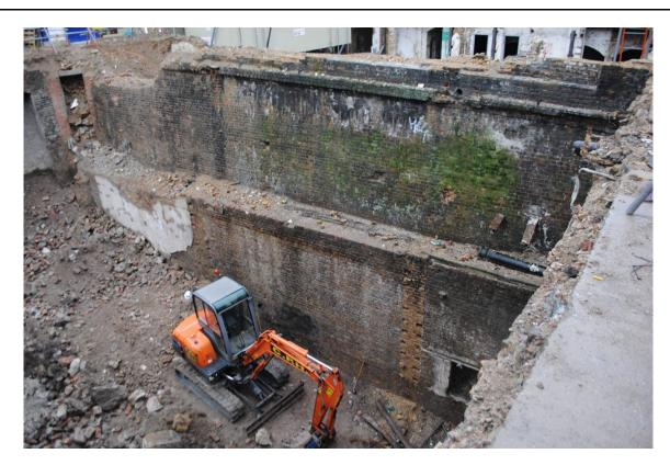
Plate 153 - Chimney and retaining walls, note void at intersection where chimney has been demolished
