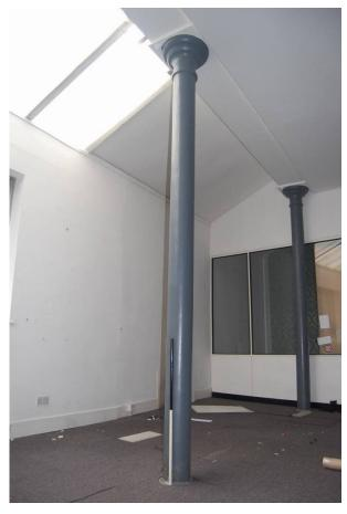
Plate 48 - 8-9 Hayne Street, cast iron column detail
