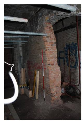
Plate 119 - 3 Lindsey Street, partially blocked archway that originally provided access to sidings
