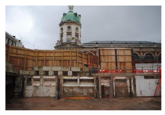
Plate 69 - 20-23 Long Lane and 22 Lindsey Street, vault detail post demolition
