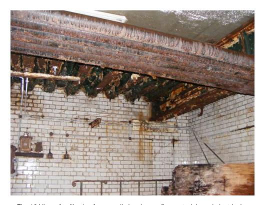
Fig. 16 View of ceiling/roof over well showing roofing materials and electrical conduits and condition resulting from severe water ingress.
