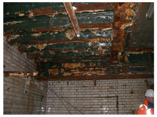
Fig. 15 View of ceiling/roof over well showing roofing materials and electrical conduits and condition resulting from severe water ingress.
