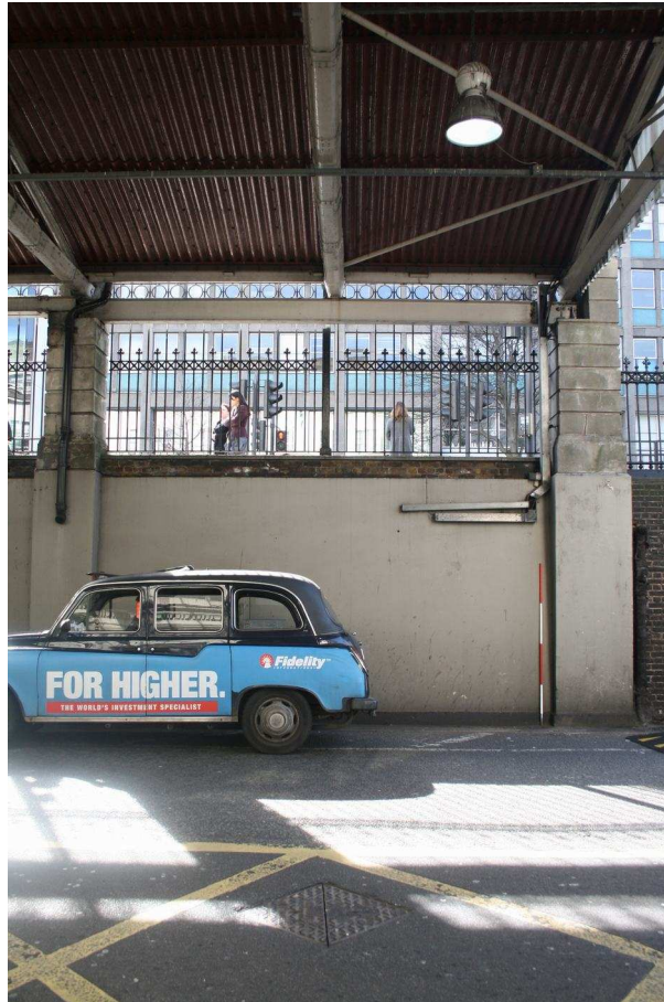
Panel 21: Central section, buttresses A and B and bay in between
