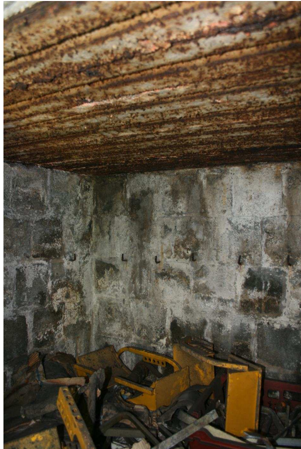
Plate 39: Interior of room A3 showing RSJ ceiling
