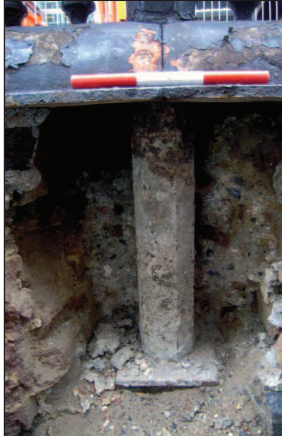
Plate 12: Exposed railing post during dismantling
