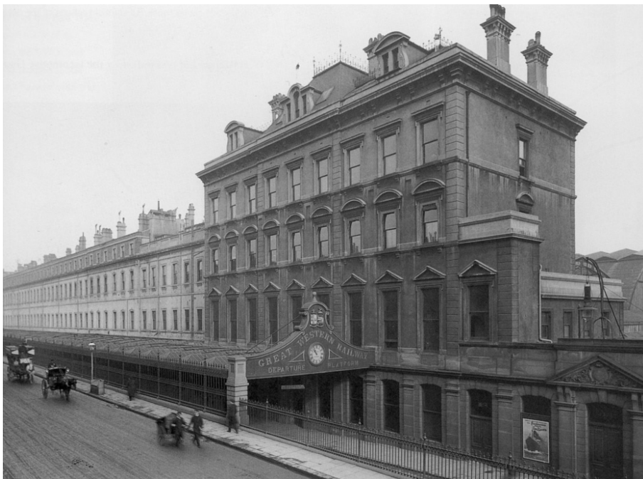
Plate 4: View of the departures road canopy, including extended area of canopy
