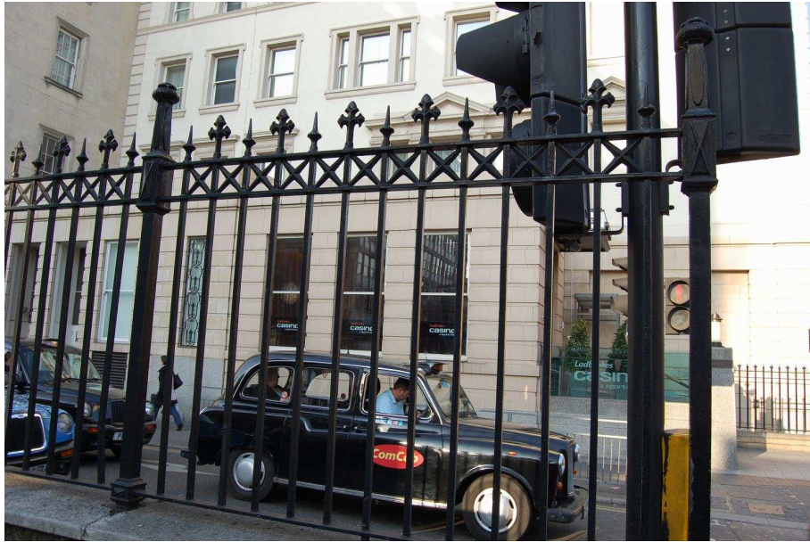
Plate 17: Eastern section, typical panel of railings
