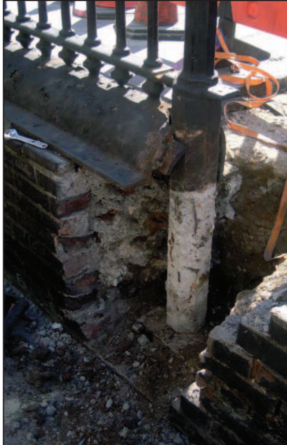
Plate 7: Exposed section of railing during demolition
