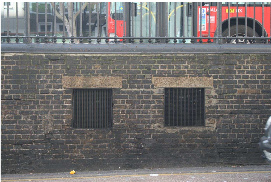
Plate 20: Recesses in western section with metal grilles
