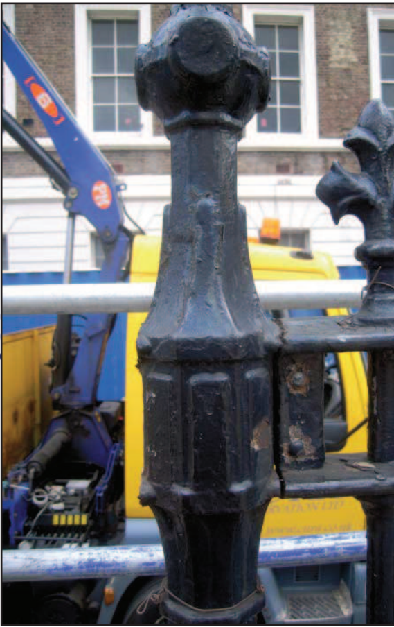
Plate 5: Railing post detail
