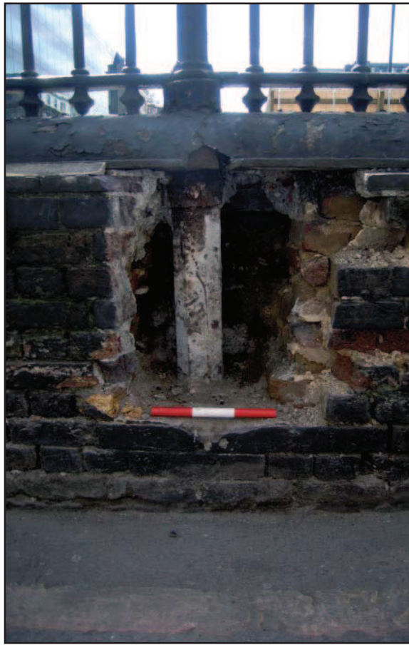
Plate 6: Exposed section of railing during demolition
