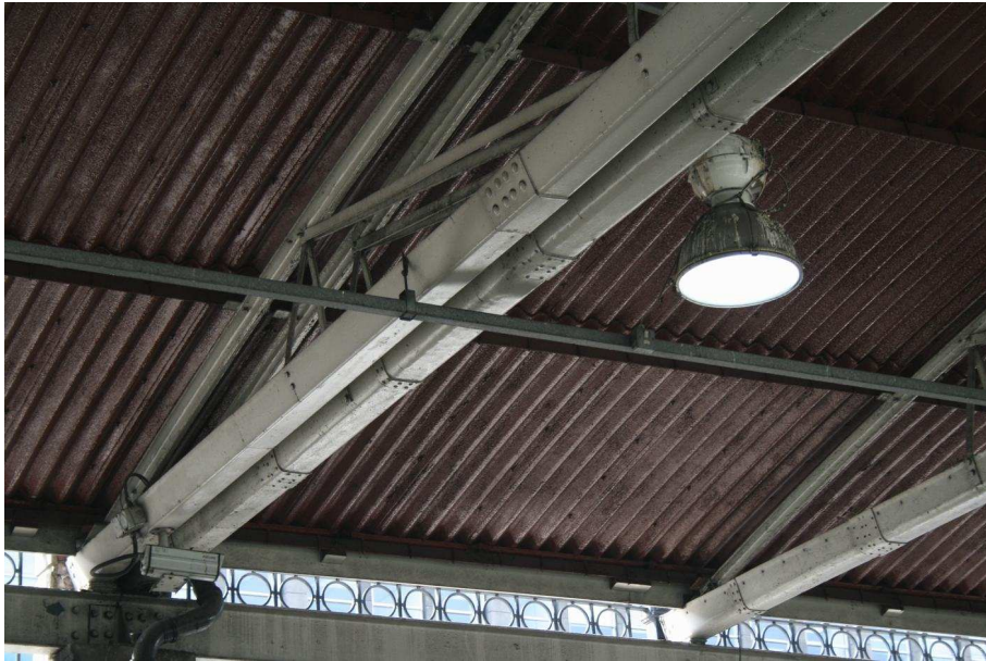
Plate 41: Detail of double truss at 8
