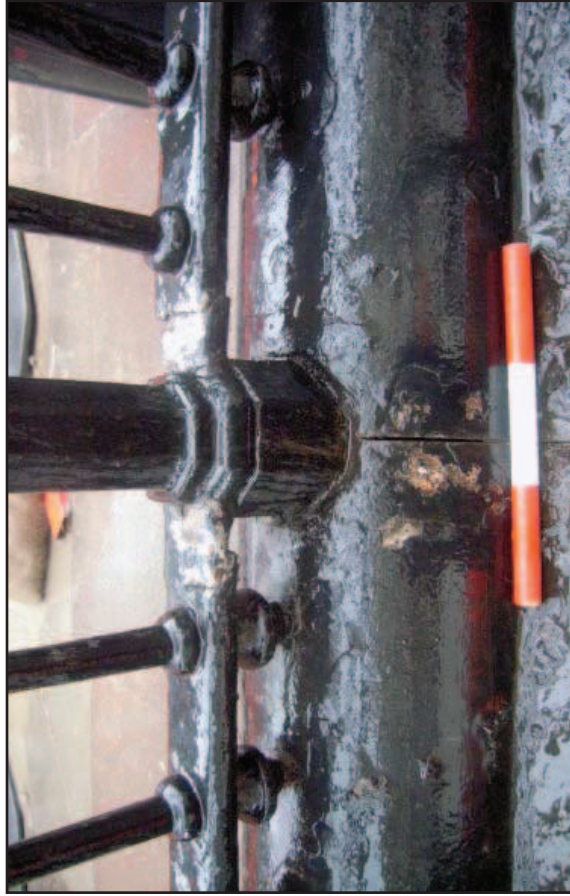
Plate 3: Railing base detail before demolition
