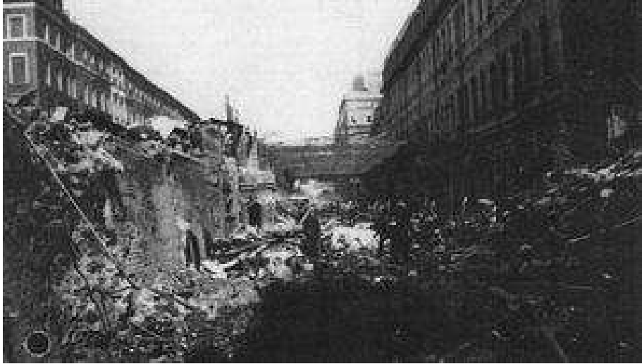
Plate 7: Bomb damage to the east end of Departures Road (Bryan 1997, 12)
