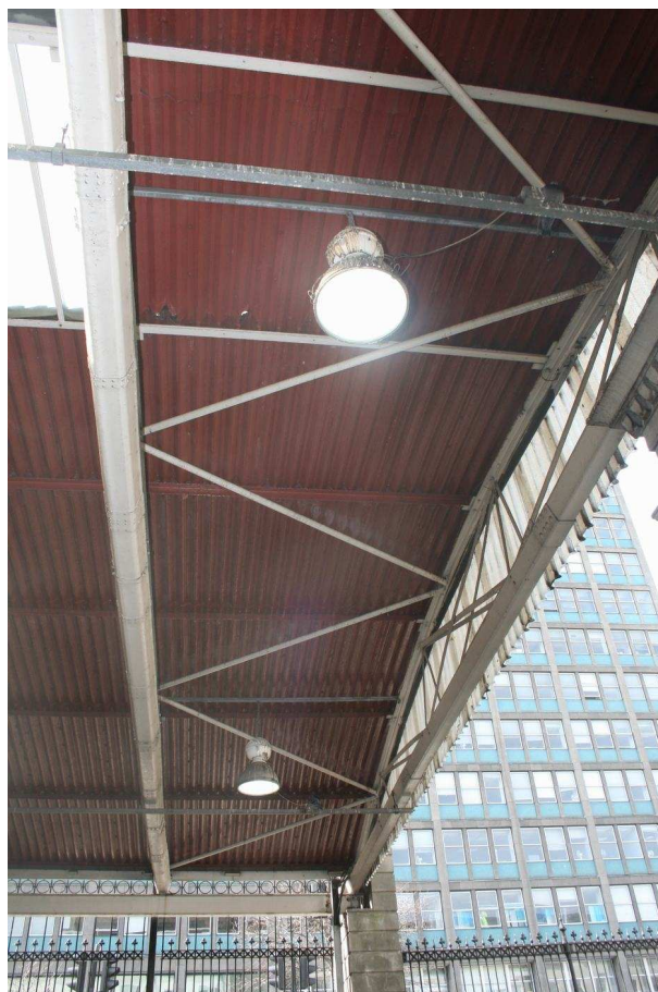
Plate 50: Wind braces between trusses 1 and 2
