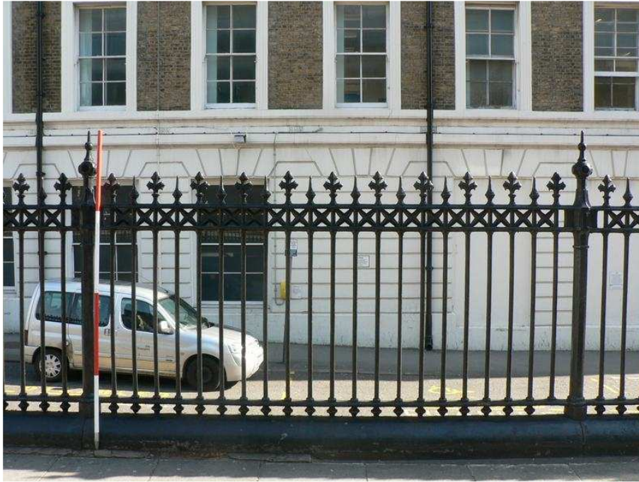
Plate 11: Original railings in the western section
