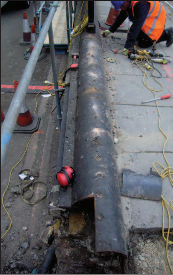
Plate 9: Cast iron railing base after removal of posts
