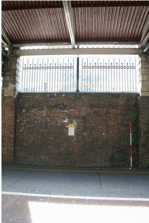
Plate 32: Buttress Q and adjoining bay to east with no dog-tooth stringcourse
