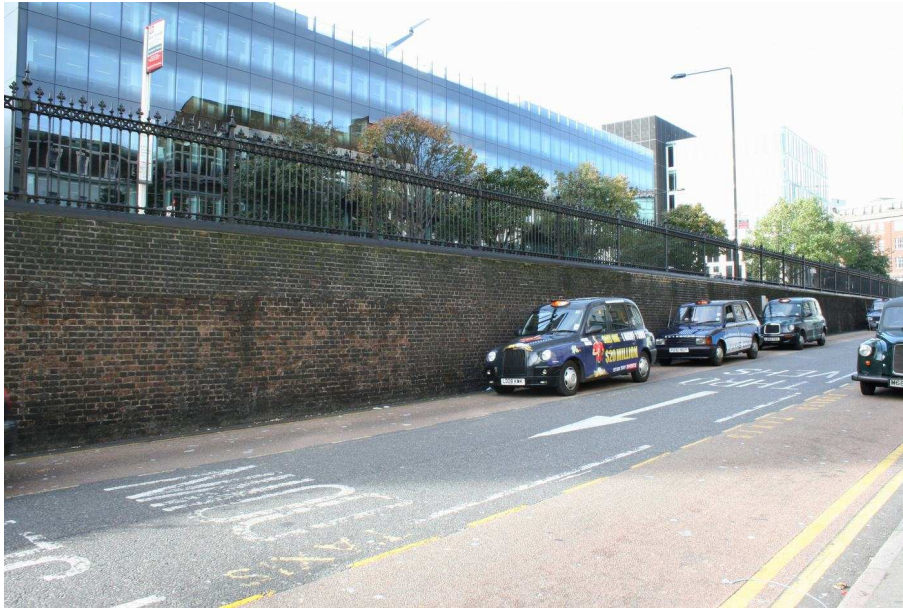
Plate 19: Western section of retaining wall
