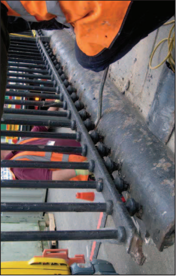
Plate 13: Section of railings during removal
