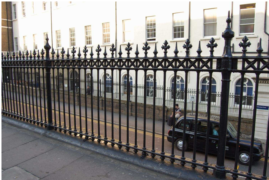
Plate 10: Cast iron base to railings in western section
