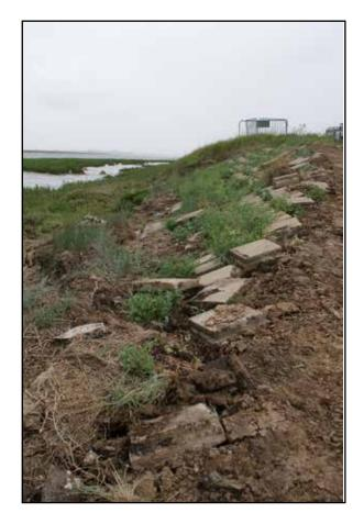
Plate 22: Breach 3. Seaward base of existing sea wall showing disturbed concrete Essex block facing and rough hewn stones along the toe of the clay bank
