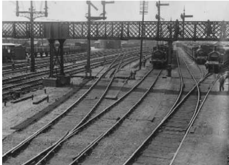
Figure 9: Ilford sidings and the main line - looking west towards Ilford station. The footbridge is visible in the first plan and was later extended. Photograph taken on 11 May 1911 (Great Eastern Railway Society collection)
