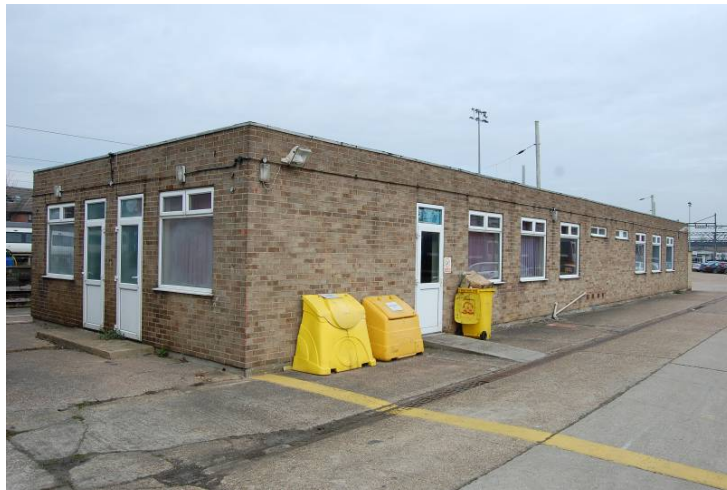
Figure 14: Bombardier Transportation Training Centre
