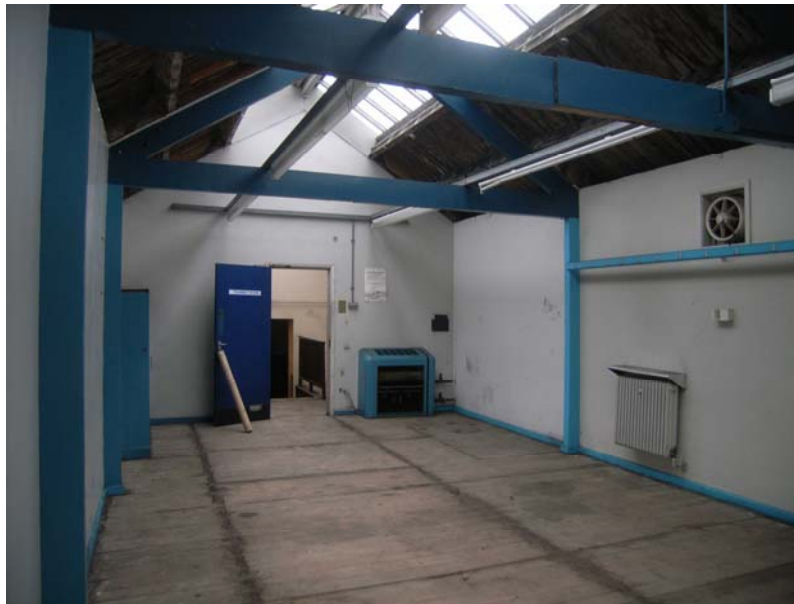
Plate 3: Interior of Building 17a
