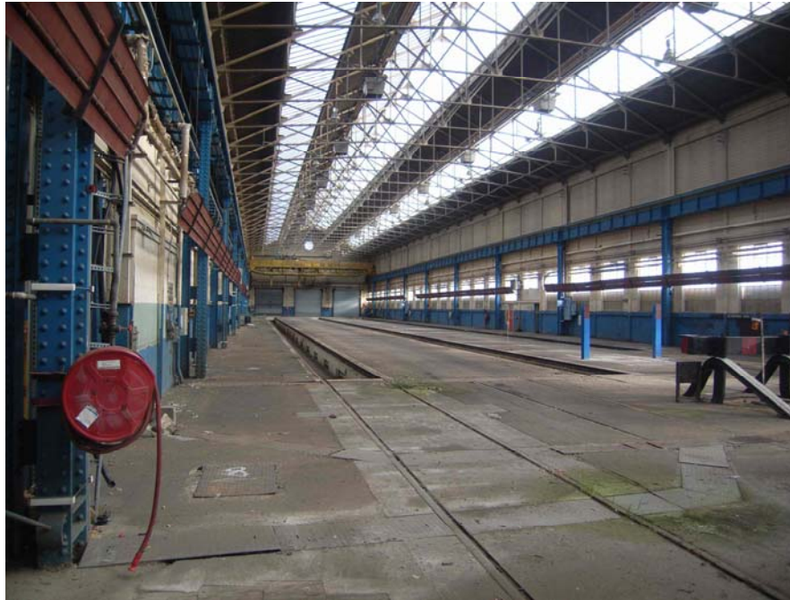
Plate 6: Interior of Building 23
