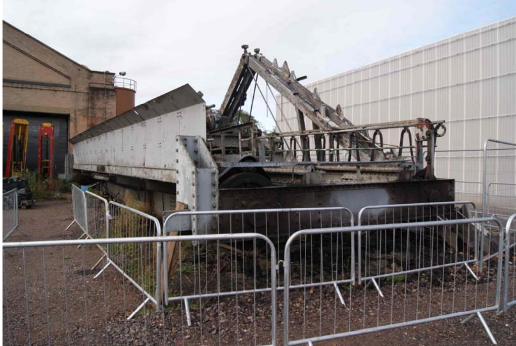
Plate 10: Salvage Item P (Gantry Crane) after salvage
