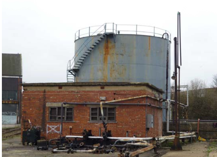
Plate 1: Heavy oil fuelling depot (Buildings 6 and 53)
