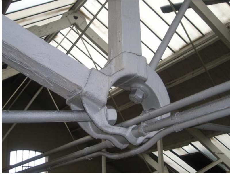
Plate 4: Roof connector in the Stores
