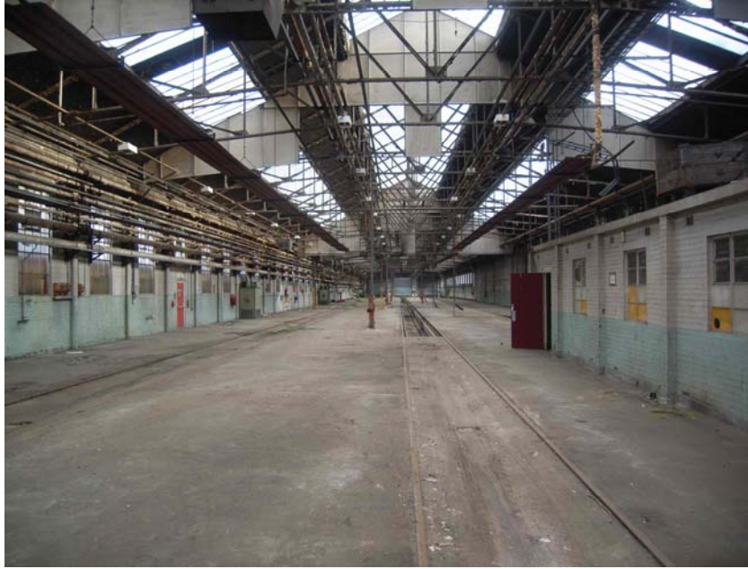
Plate 7: Interior of Building 22
