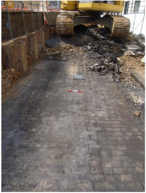
Plate 1: General character of wooden sett roadway seen in top of Basement Clash Trench looking towards the northwest
