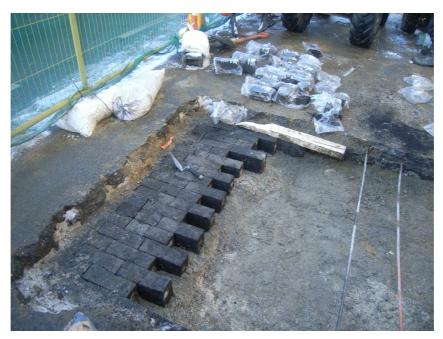
Plate 5: Relaying of setts after initial trench investigations TPSW3
