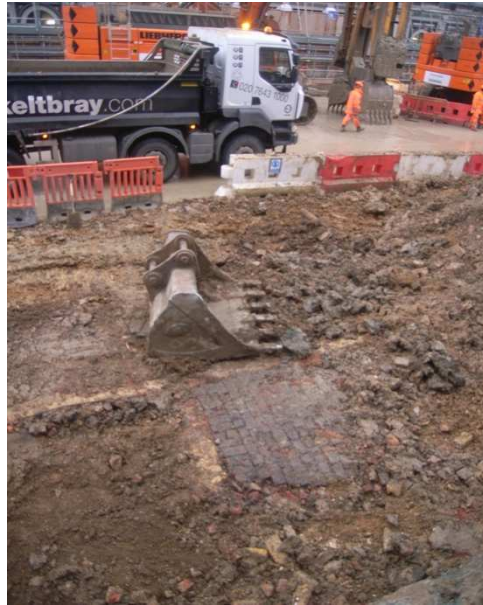
Redbrick floor (6545) of cellars (6546) beneath southern edge of Eastbourne Terrace. Looking north
