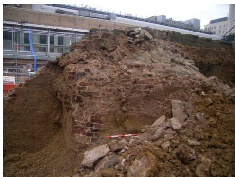
Demolition of retaining wall between Eastbourne Terrace and Departures Road
