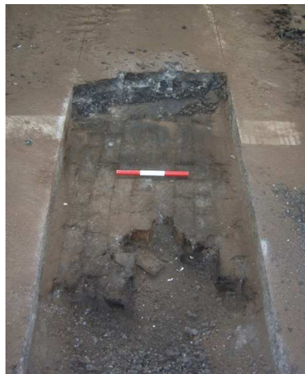
Decayed section of setts
