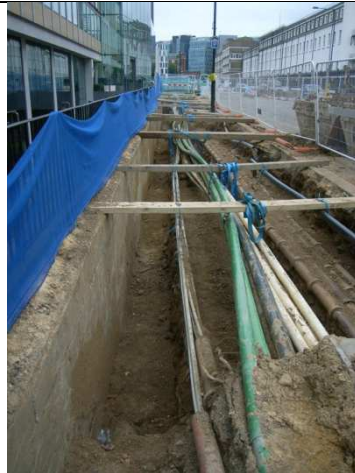
Utilities Trench 1. Looking west. Wall 6004 is on the left
