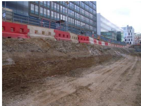
Side of brick built Sewer (6133) looking northwest
