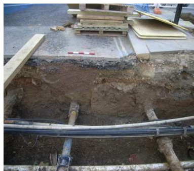
Utilities Trench 1 – Section opposite Cleveland Terrace
