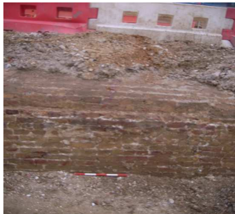
Side wall and top of Sewer (6133) looking south
