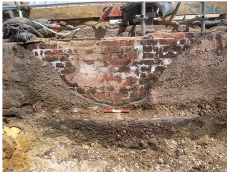
Upper bricks 6427 and lower concrete footings 6410 of Macmillan House Basement
