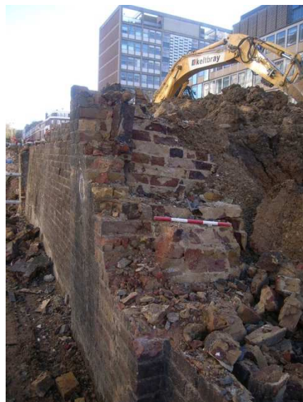
Demolition of retaining wall between Eastbourne Terrace and Departures Road
