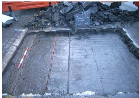
Wooden roadway at eastern end of Departures Road. Looking east. Showing seam where setts were lifted to build basement of Macmillan House
