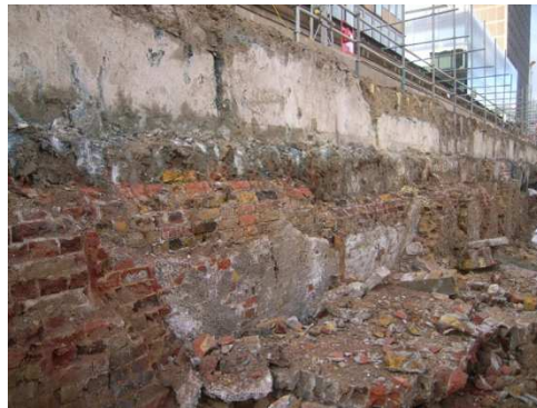
Second inner cellar wall added to inner face of original white washed southern wall of cellar (6546)
