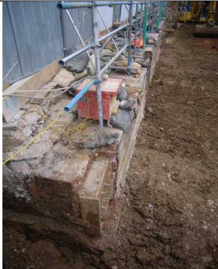
Corner of Macmillan House Basement
