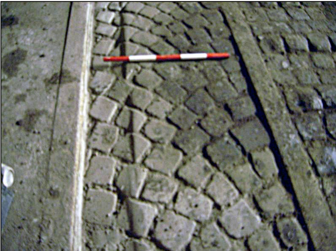
Plate 24: Worn linear groove in the cobbled surface of Milk Ramp. A iron rail is to the right
