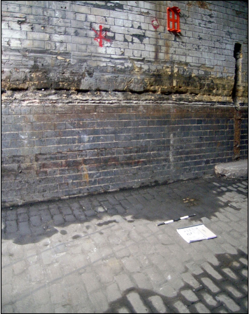
Plate 27: Overall View of Wall
