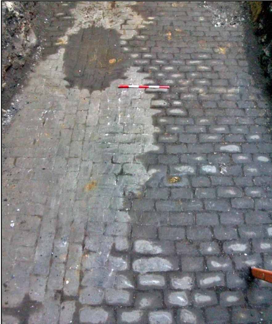
Plate 16: Surface 2065 showing drainage gully
