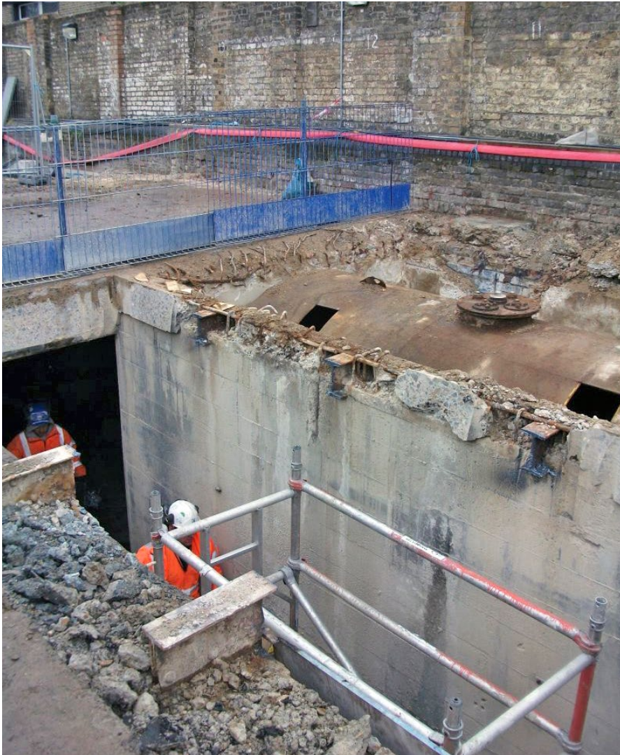
Plate 25: Petrol tank and bund wall truncating the Milk Ramp during dismantling
