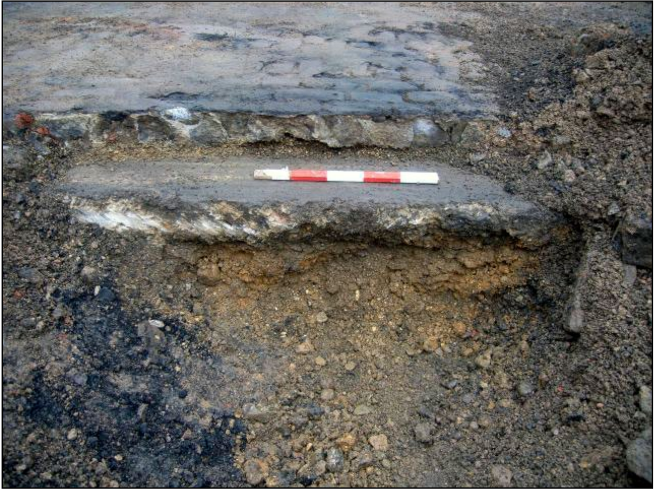
Plate 11: Surface 2011, close up section. Looking north-west
