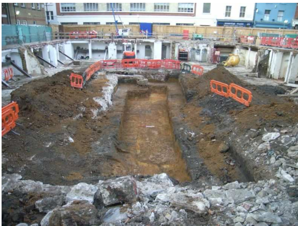
Plate 15: Uneven nature of the quarrying, looking west
