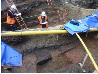
Working Shot of Grout Shaft 5 excavations, looking W
