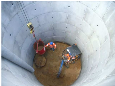
Grout Shaft 1, natural gravels 5501
