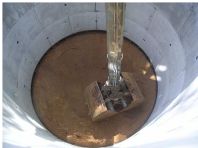
Grout Shaft 2, natural deposits, mid depth
