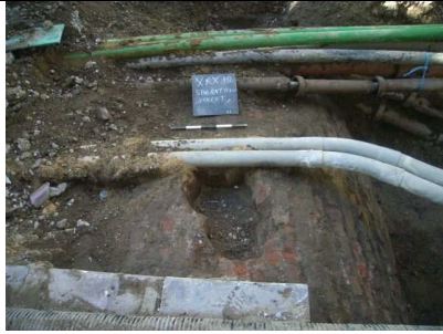
Cellar 5491 looking north, showing "coal hole," cut into cellar roof
