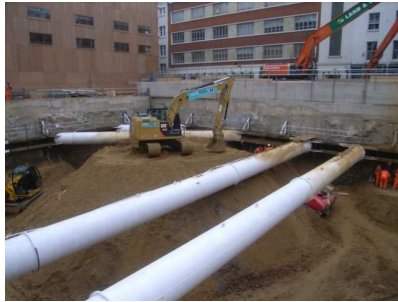
General view of bulk dig, looking SW
