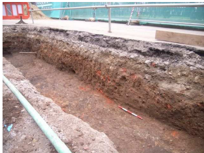
Grout Shaft 2, upper deposits, looking SE
