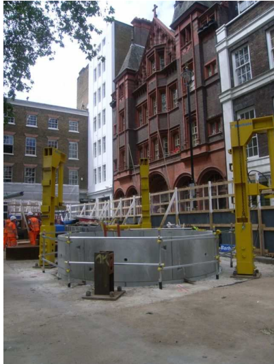
Grout Shaft 2, general view, looking NW
