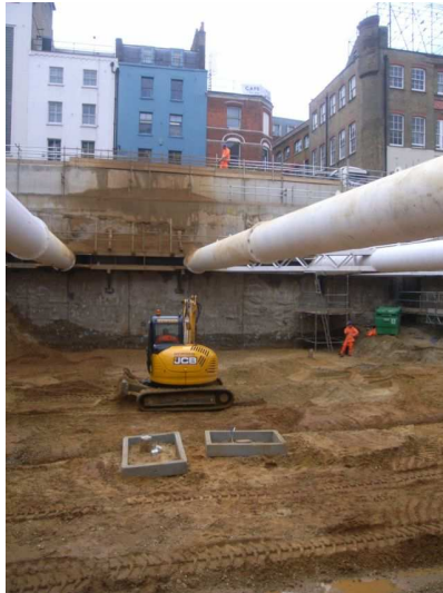
General view of bulk dig, looking west
