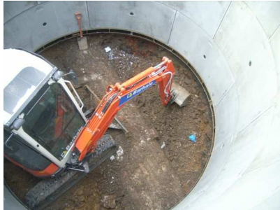
Grout Shaft 1, barrel vaulted sewer
