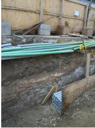
Great Chapel Street, wall
