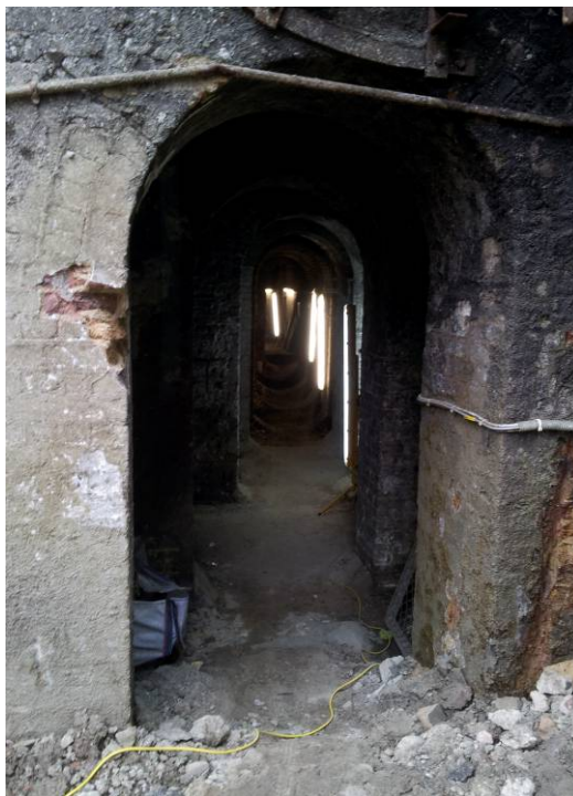
Fig 5 The eastern entrance into the Shunters' Rooms, looking west
