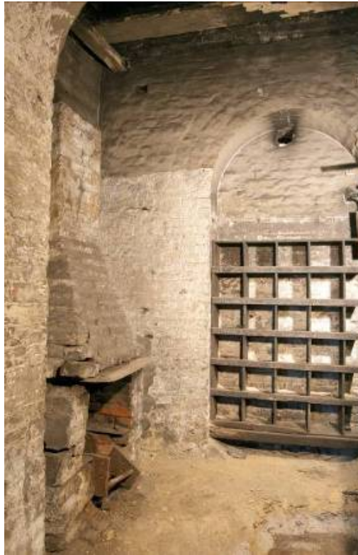
Fig 6 View of the eastern fireplace and infill (Room 3), looking west
