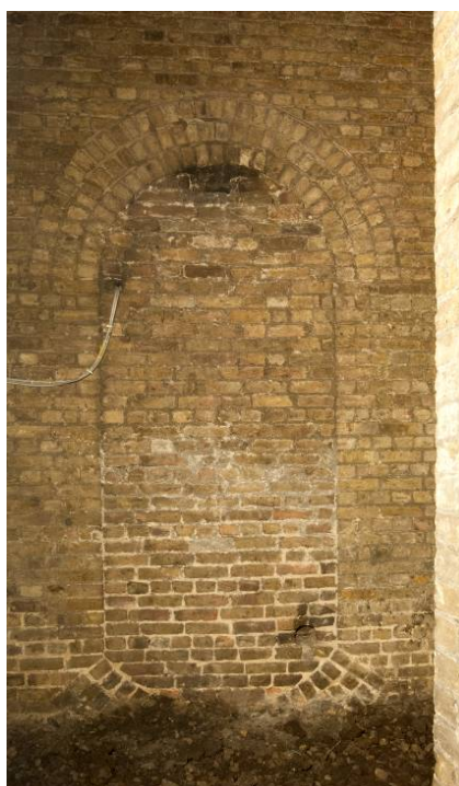
Fig 9 The infill, looking east
