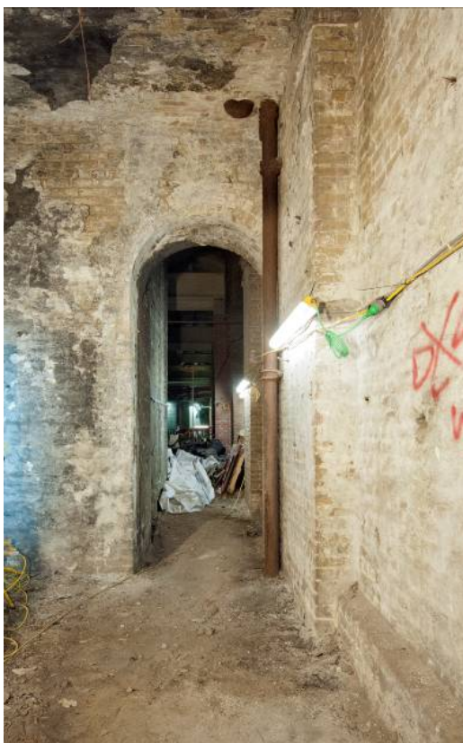
Fig 12 The corridor to the west of the west of Room 9
