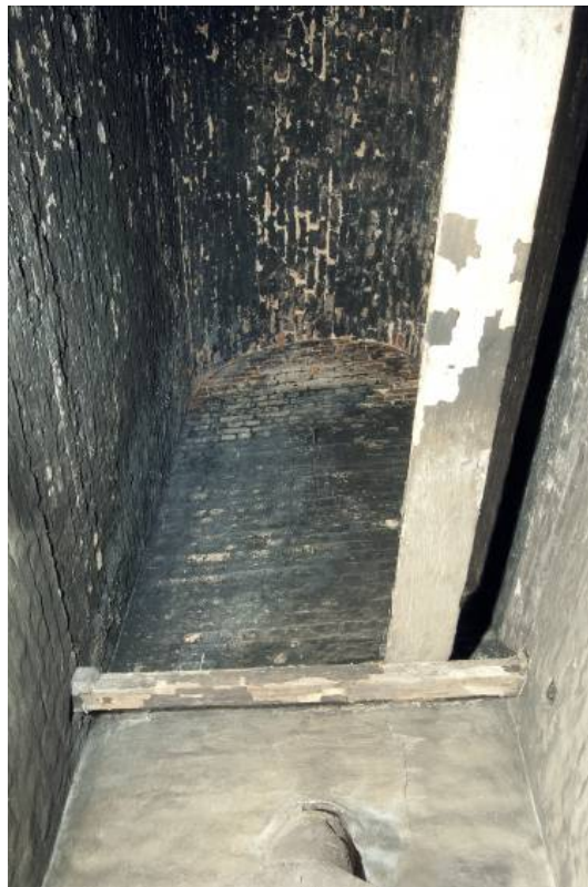
Fig 7 Detail of the barrel vault above the eastern fireplace
