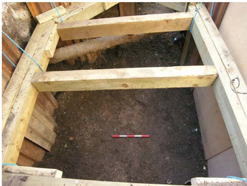
Photo 1, Targeted watching brief at formation level of 1.7m bGL, looking south-west.
