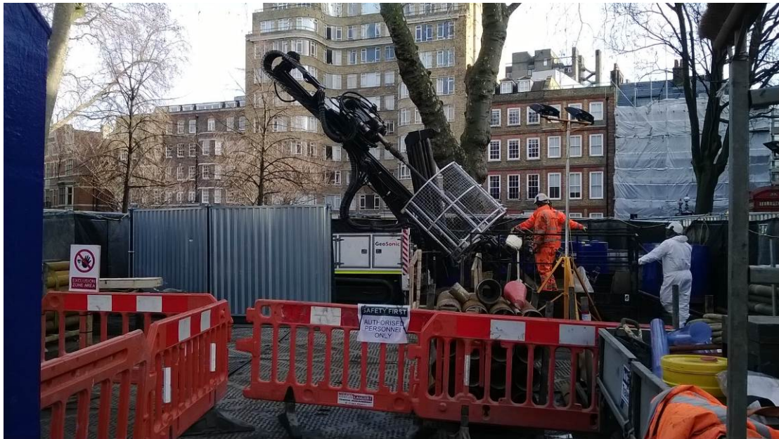
Photo 1 Showing Borehole drilling rig, drilling Borehole at 45° angle, looking east
