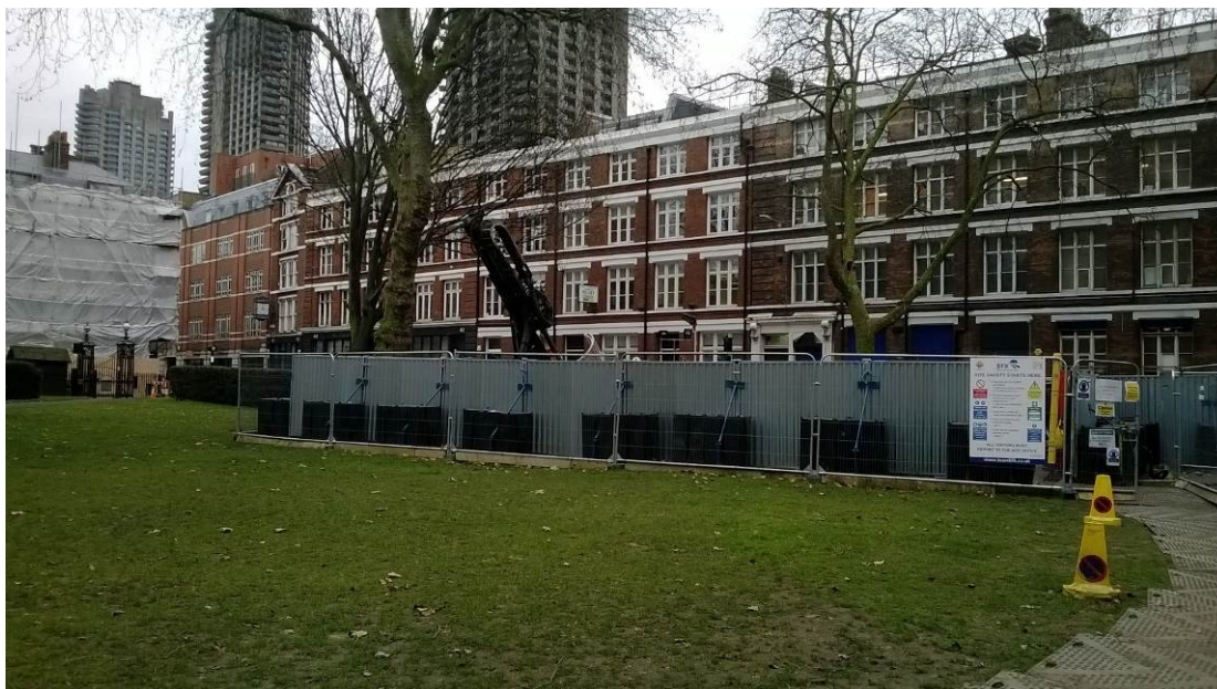
Photo 2 View of site showing area of borehole drilling works, looking south-east
