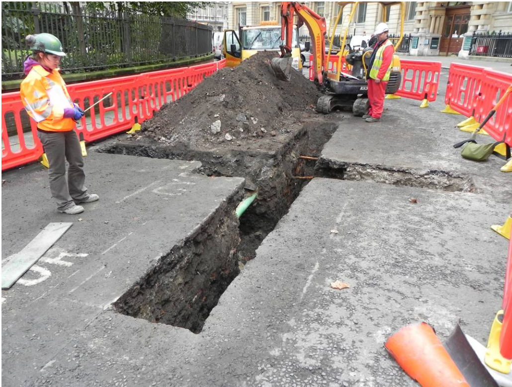
South facing: Finsbury circus Western Grout shaft
