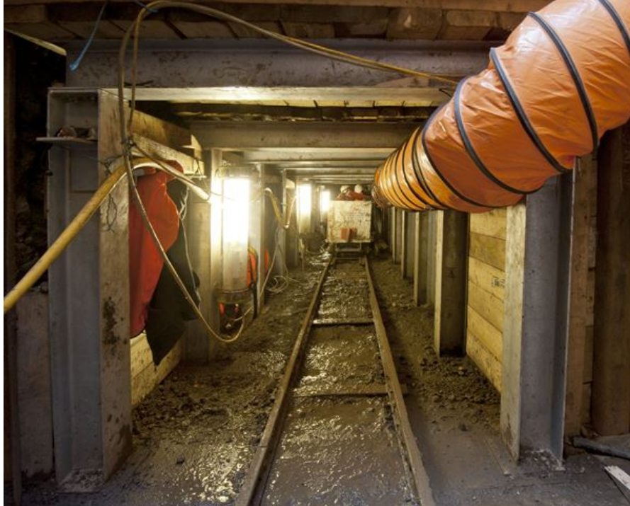
Photo 15: The MHS2-100 sewer heading; looking south-west
