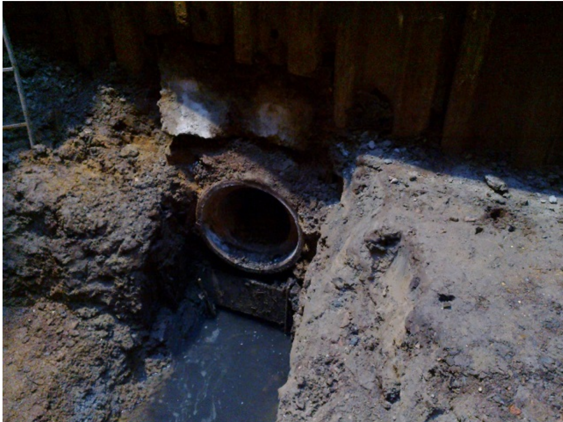
Photo 18: River clay and gravel bands overlying natural terrace gravels, truncated by Manhole X and heading
