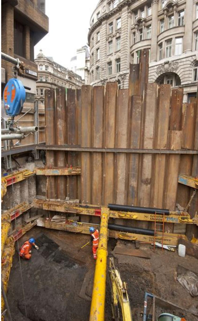
Photo 4: MHS1 excavation, looking west
