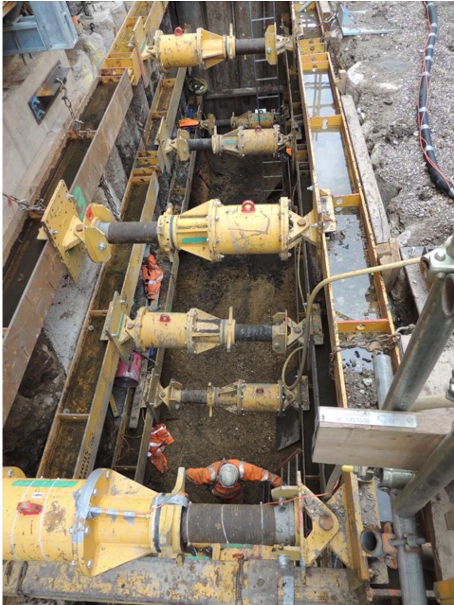
Photo 1: Excavation in Utilities Corridor GL8–QVT, looking west
