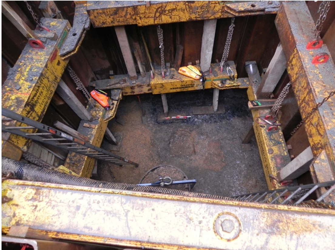
Photo 19: View into MHS2, looking down to south
