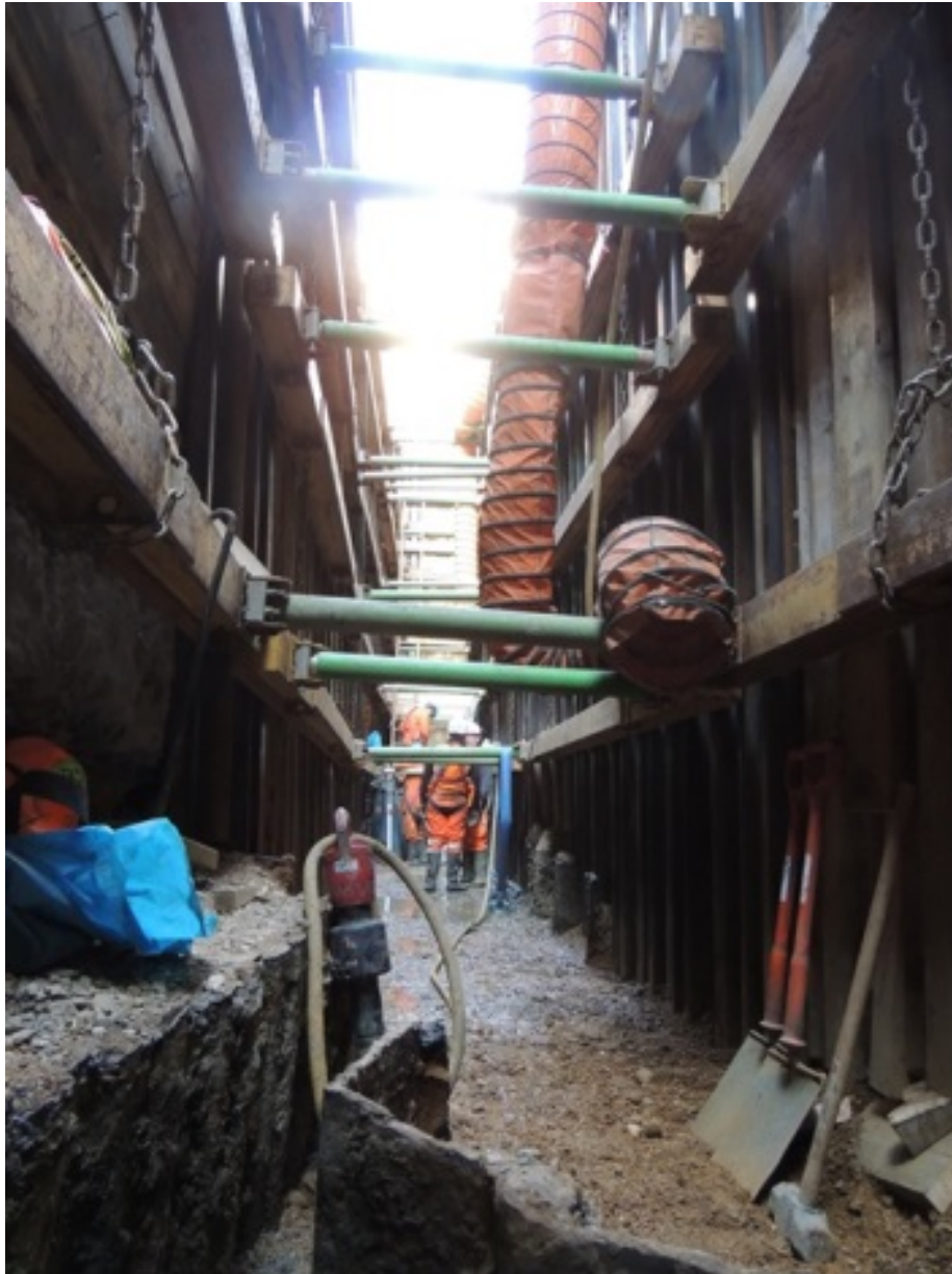
Photo 7: Open Cut Sewer, looking east
