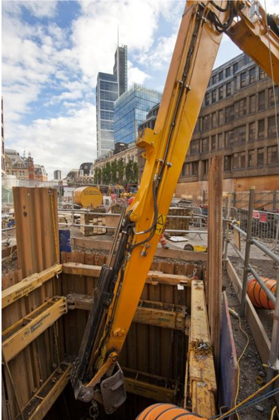
Photo 10: Lifting up the skip in MHS2-100; looking east
