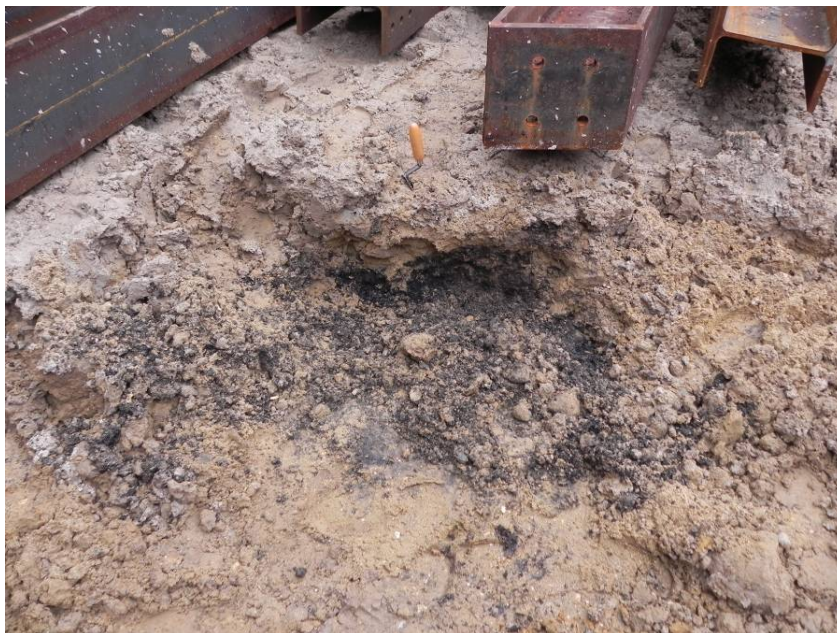
Photo 2, OSD trench, 19th-century dump deposit [40], looking north-west.
