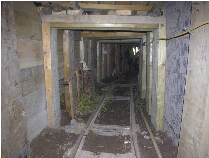
Photo 1 London Wall heading shaft, looking west
