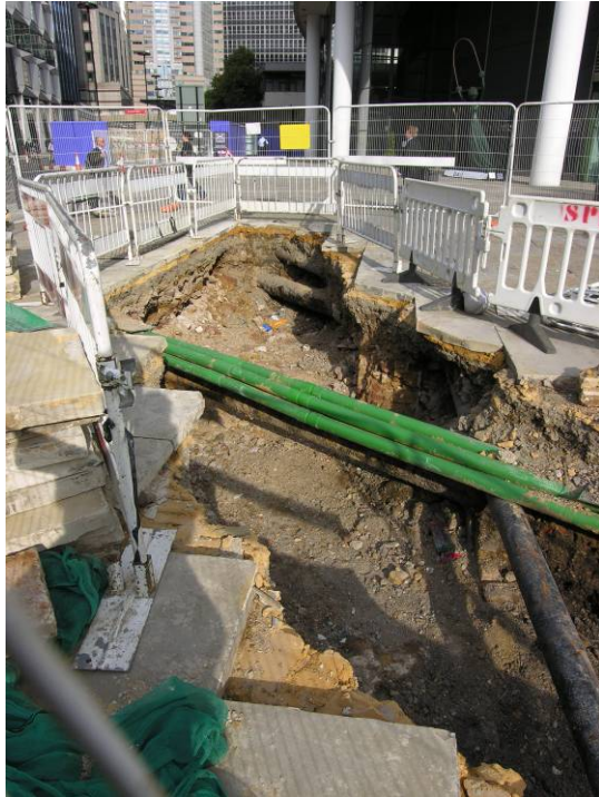
Photo 6, London Wall, looking west
