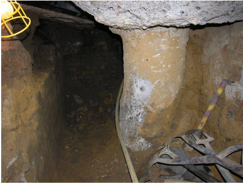
Photo 4 Excavated tunnel approximately mid way between western and eastern access shafts. Modern foundations truncating earlier stock brick wall, looking east
