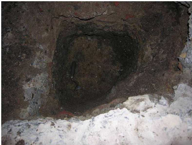
Photo 11 Sandy Concrete footing for existing basement at 0.9m bGL, looking south
