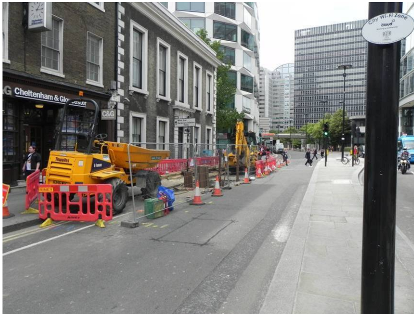
Photo 3 Location of Trench 1 on London Wall (centre), looking south-west.
