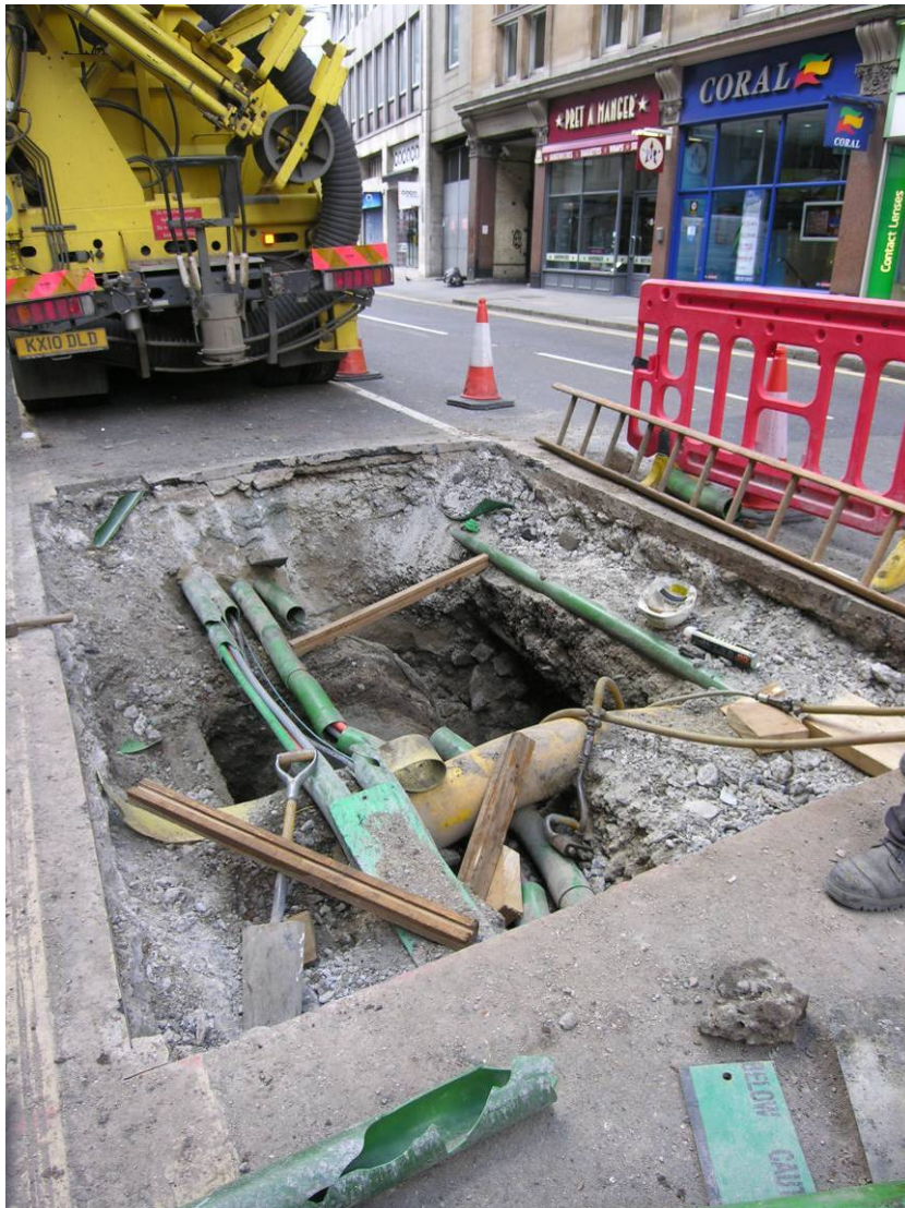
Photo 5 Location of Trench 2 on London Wall, looking north-west.
