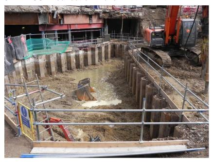
Photo 1 OSD trench, after removal of 0.5m of piling mat, at 108.90m ATD, looking north
