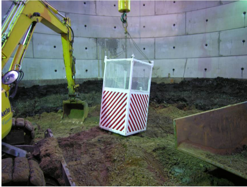
Photo 1 Access to the shaft was via a manrider cage.
