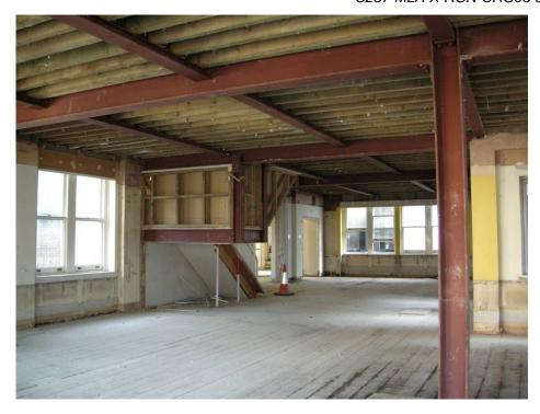
Fig 38 Ceiling joists in westernmost room, on Blomfield street, looking east
