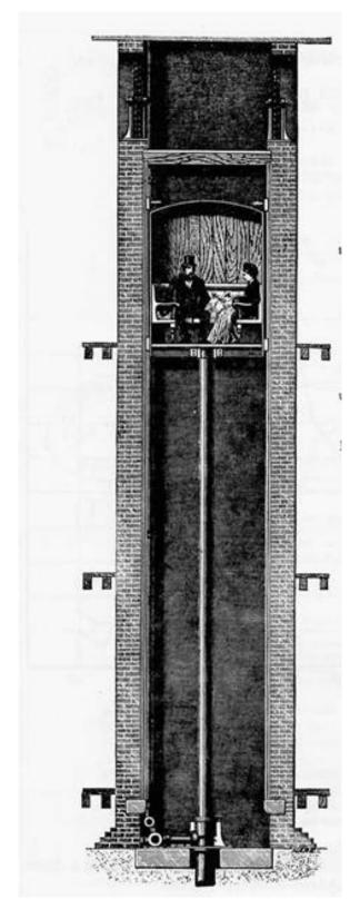
Fig 37 A Direct acting hydraulic lift c1870–80 (Image from Charles Sturt University)
