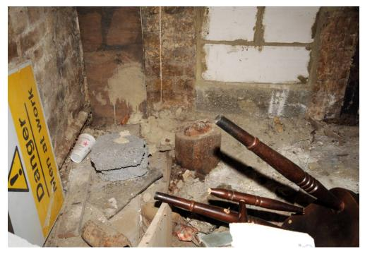
Fig 31 The surviving stump of the direct acting hydraulic lift piston beneath the geometric staircase, lower ground floor level looking west
