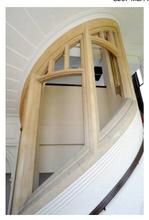
Fig 28 The decorated stonework of the geometric staircase, looking south
