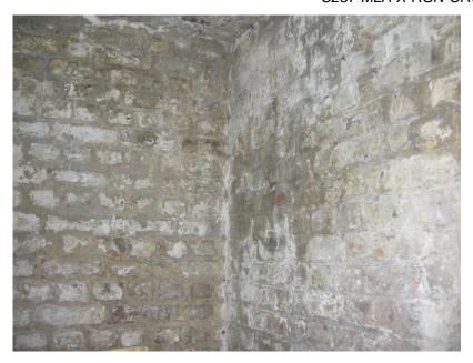
Fig 54 Straight joint between trackside wall and later room partition, in second room from east, looking west
