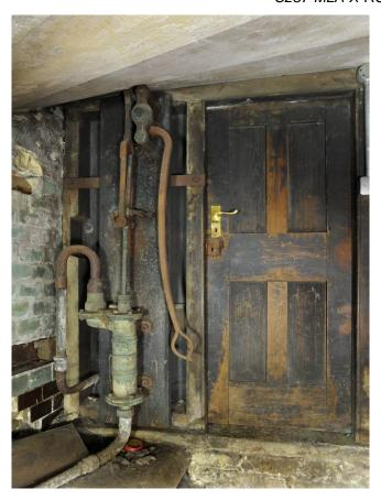
Fig 32 The hydraulic hand crank, below the geometric staircase, lower ground floor level looking west
