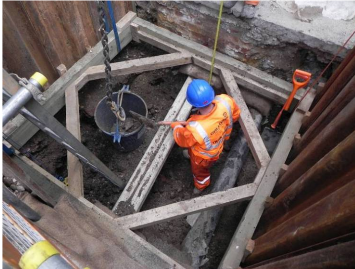
Photo 9: Pit 2 – Galldris excavate 19th and 20th-century utility and construction backfills, looking south-west.
