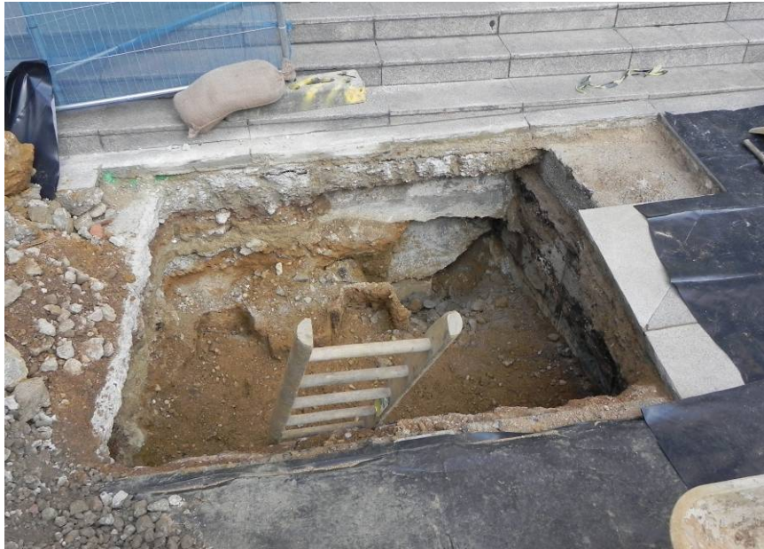
Photo 24: Trench 15 – Excavated by Galldris to c 112.80m ATD (1.2m bGL), concrete walls top and right, looking north.
