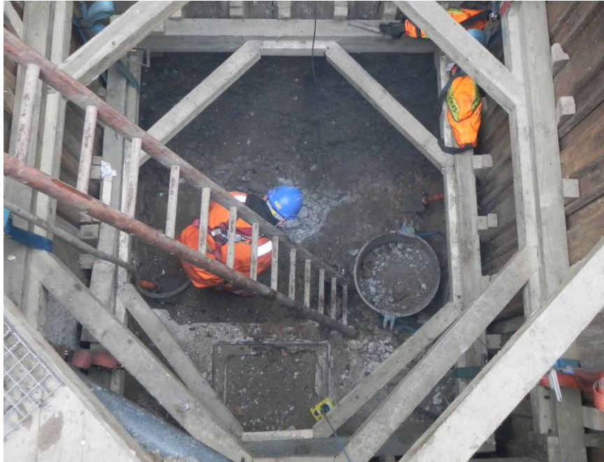
Photo 8: Pit 1 – Concrete wall foundation slab being broken out at 108.59m ATD (3.70m bGL), with a concrete backfilled manhole (centre bottom), archaeological deposit [901] (top right), south at top.
