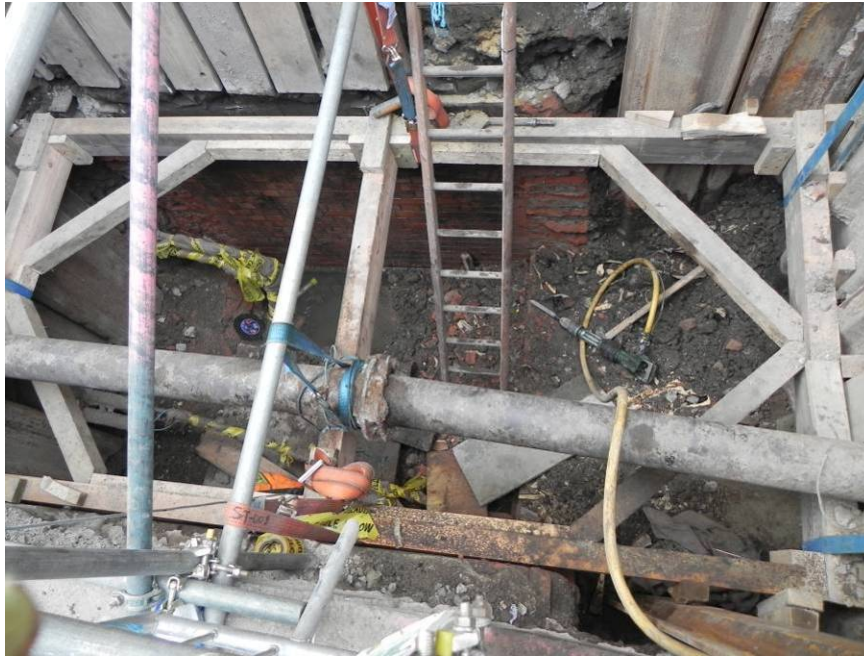
Photo 15: Pit 9 – Excavated to a depth c 3.00m bGL, with modern utility structure brick walls (centre and left) and construction backfill (right), looking south.
