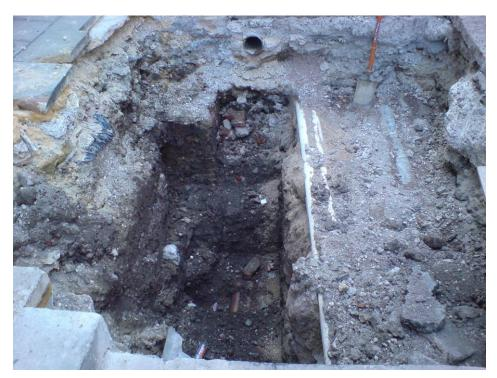
Photo 10: Trench 1a – Gas pipe (right) and telecommunication cables (white pipes), with a deeper utility trench (ceramic pipes) truncating the south half of the trench (centre and left)(looking west).
