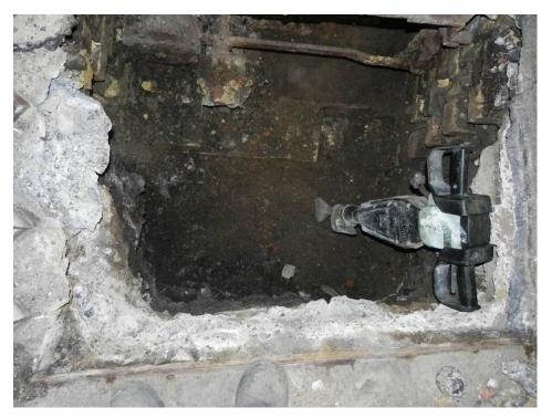
Photo 22: Railway Tavern Trial Trench - Foundations of the Railway Tavern with to 19th-century walls, disused machinery, and construction backfill (north at top)
